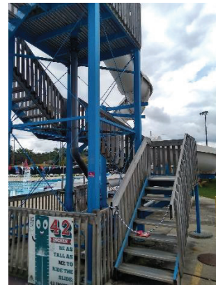
3" X 1½" STEEL TUBE AT LANDING (TO BE REPLACED)
