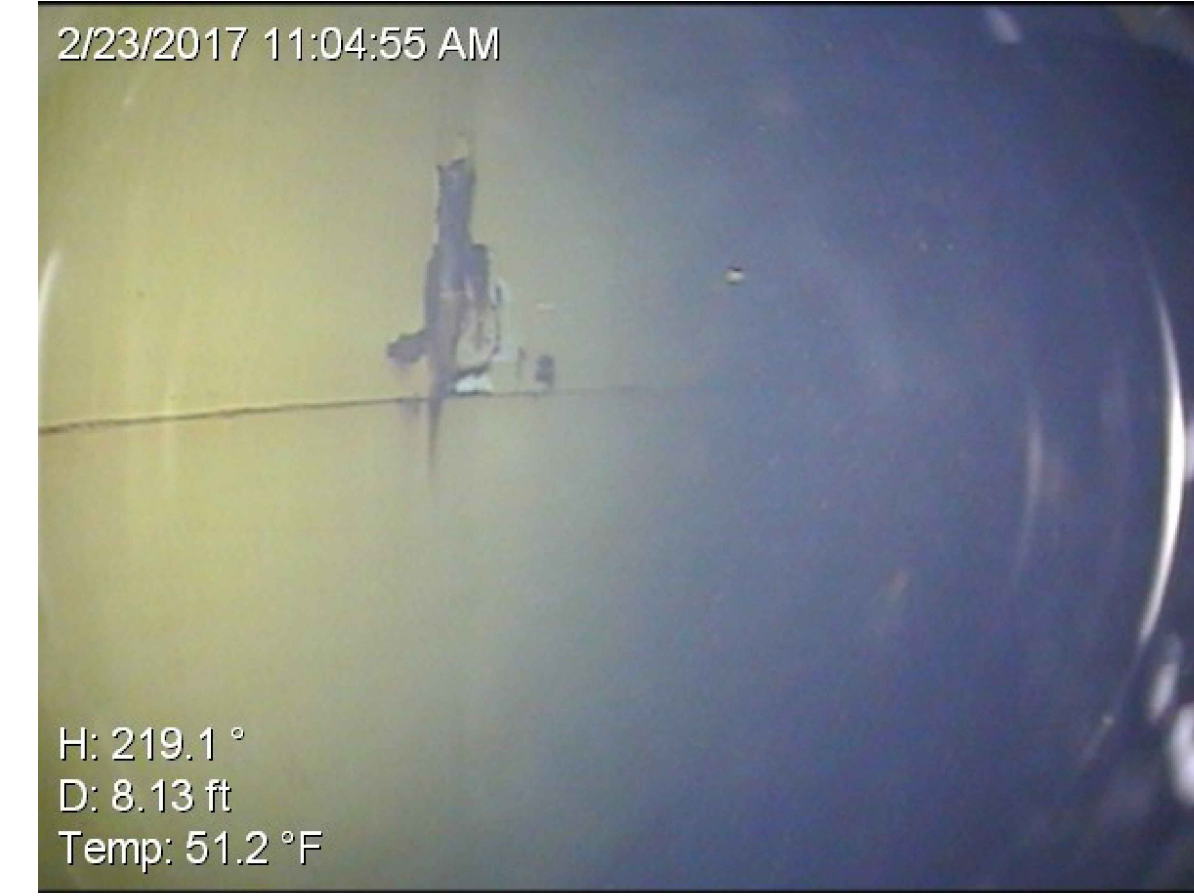
WET INTERIOR COATING-SIDEWALL LOCATION 2 ON C-102
