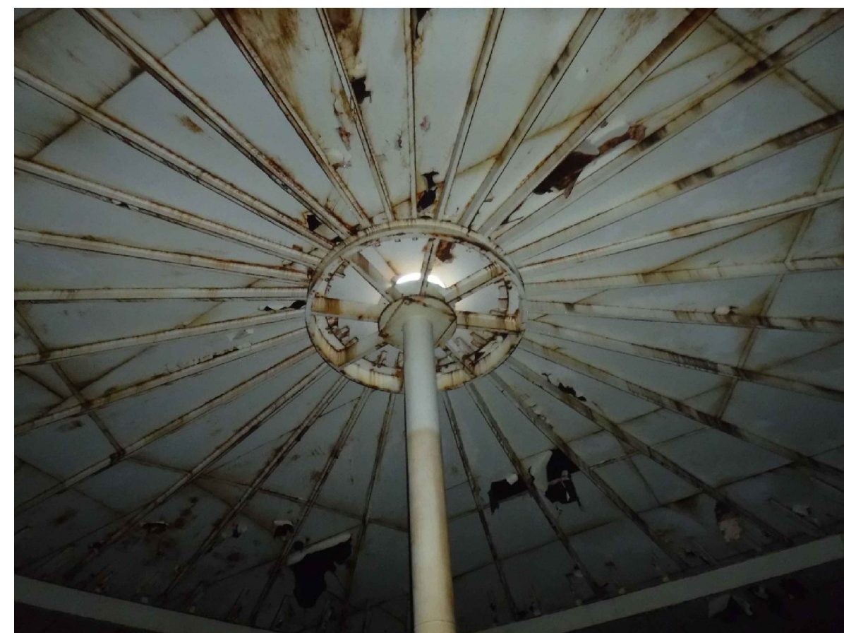
WET INTERIOR COATING-ROOF LOCATION 1 ON C-102
