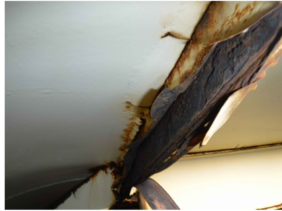
MISCELLANEOUS STEEL REPAIR-WIND GIRDER REPLACEMENT LOCATION 5 ON C-102
