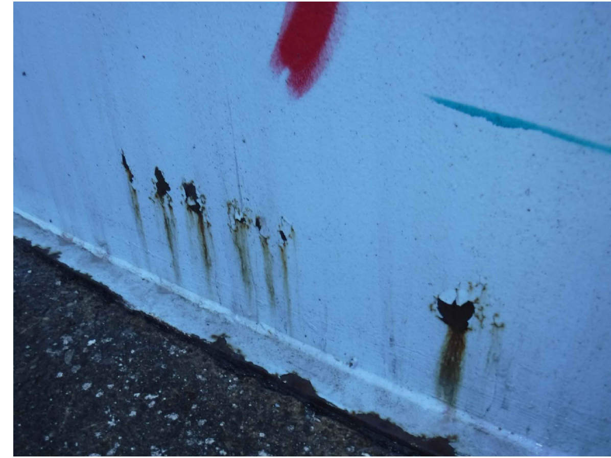
EXTERIOR OVERCOATING-LOWER SIDEWALL LOCATION 6 ON C-102
