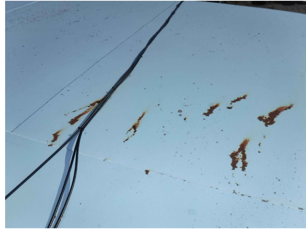
EXTERIOR OVERCOATING-ROOF LOCATION 6 ON C-102
