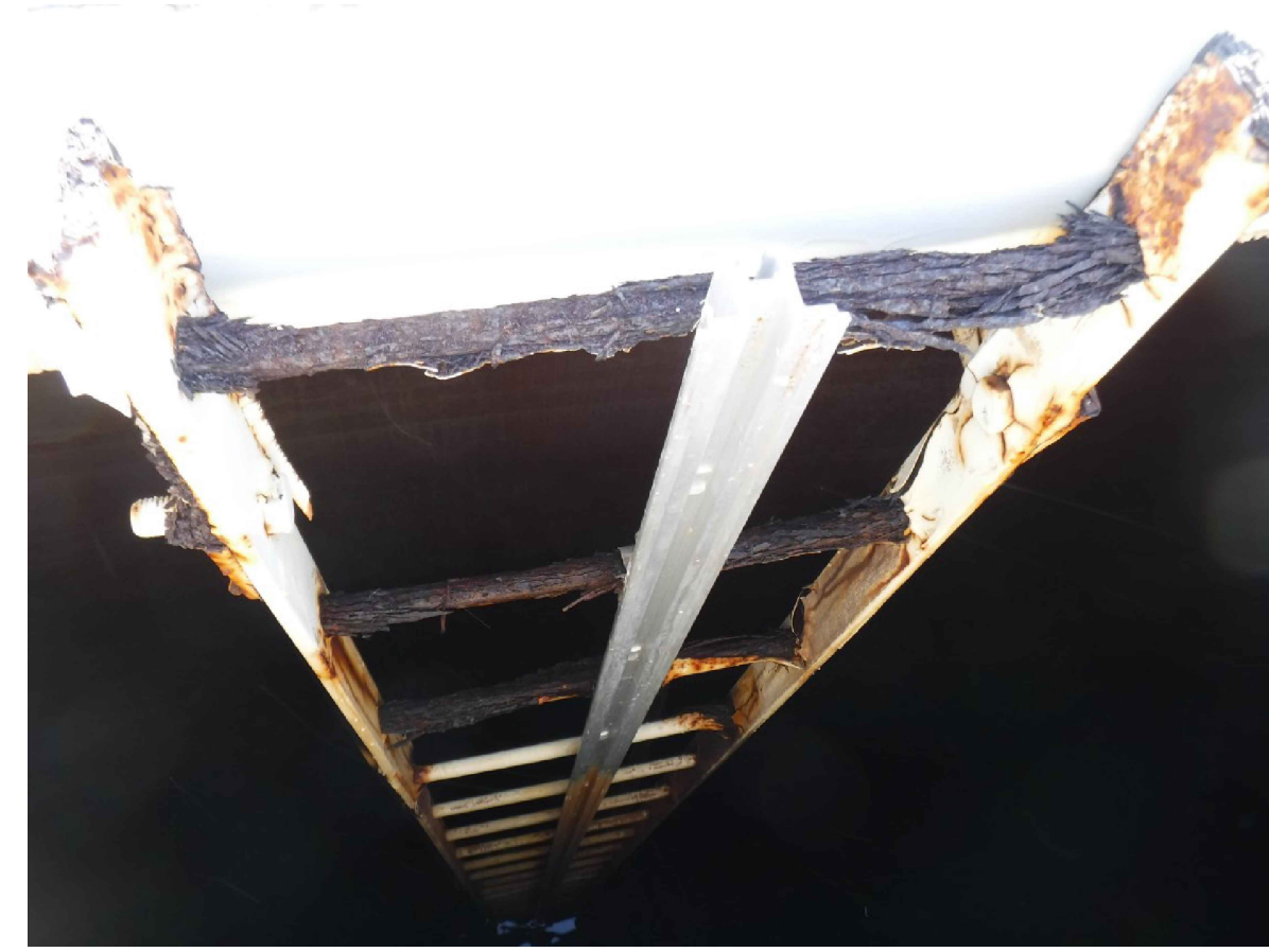
WET INTERIOR LADDER-CORRODED RUNG REPLACEMENT LOCATION 4 ON C-102
