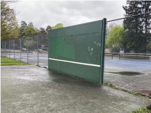
PRACTICE WALL / COURT ACCESS
