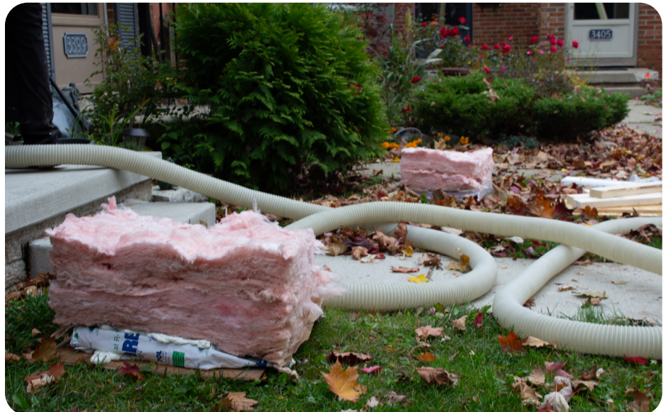
Photos of work underway at Colonial Square.
