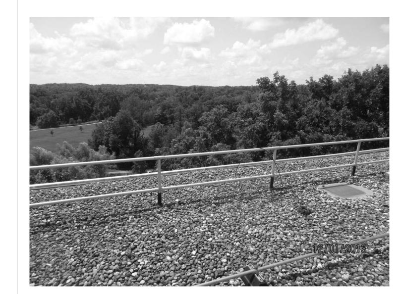
ROOF MOUNTED GUARDRAILS
