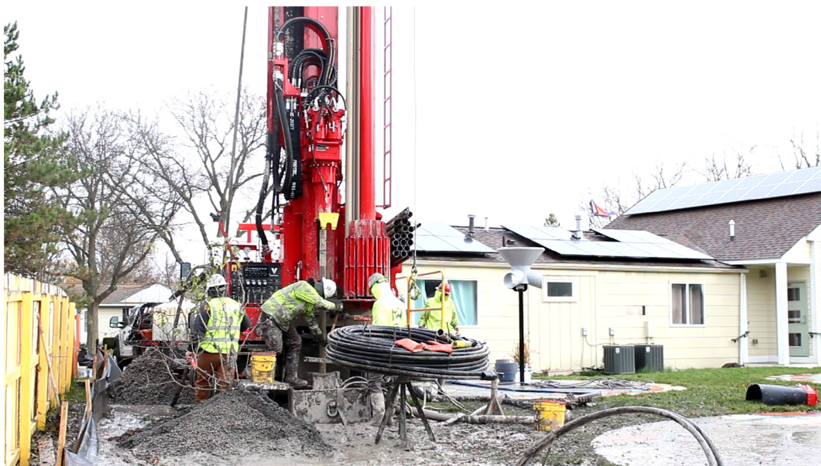
Drilling for the geothermal system at the Bryant Community Center.
