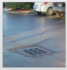
Runoff from coal-tar-sealcoated pavement goes down storm drains to receiving water bodies. The runoff contains high concentrations of PAHs and related chemicals that can harm aquatic life.<sup>16</sup>
