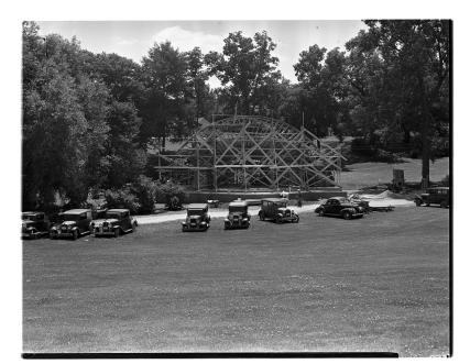
to shine on the performers. They started by building the foundation out of concrete blocks, then they framed the arc and back out of wood and covered them in concrete. They used wooden supports and scaffolding for the work. They gave the structure a composite roof in a nice copper color. You can find some pictures of the bandshell construction below.
