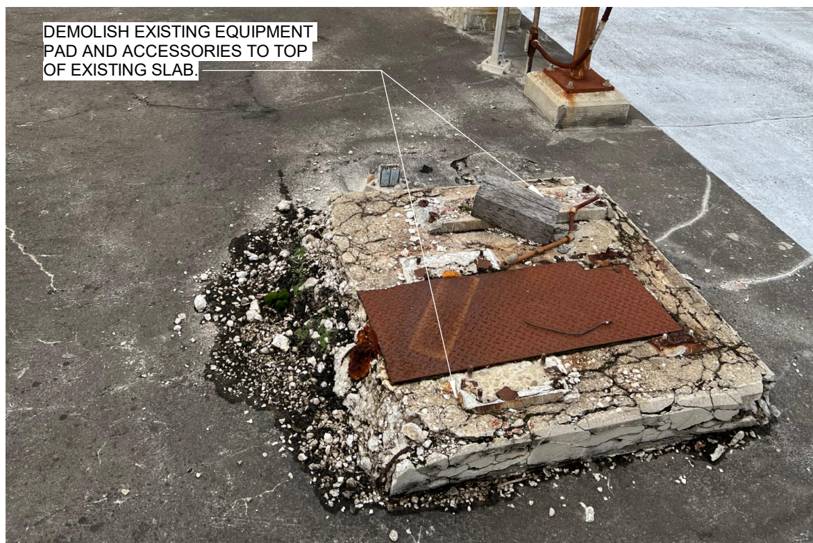
DEMOLITION DETAIL EXISTING CONCRETE PAD SCALE: NOT TO SCALE
