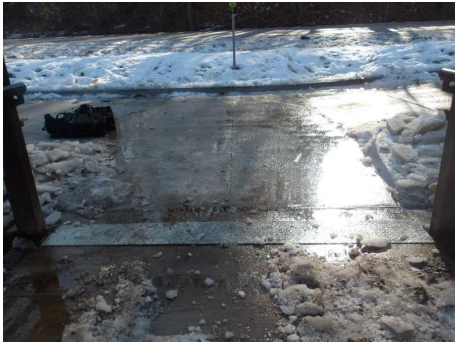
Photo 6 – New South Approach (Looking South)
