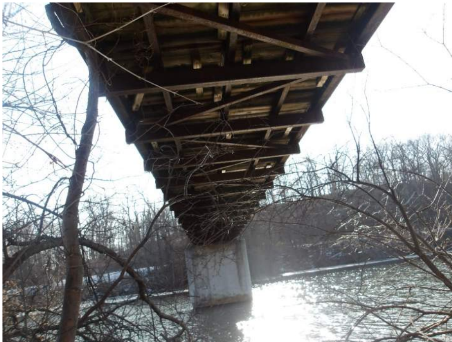
Photo 20 – Deck Underside Span 3 (Looking South)
