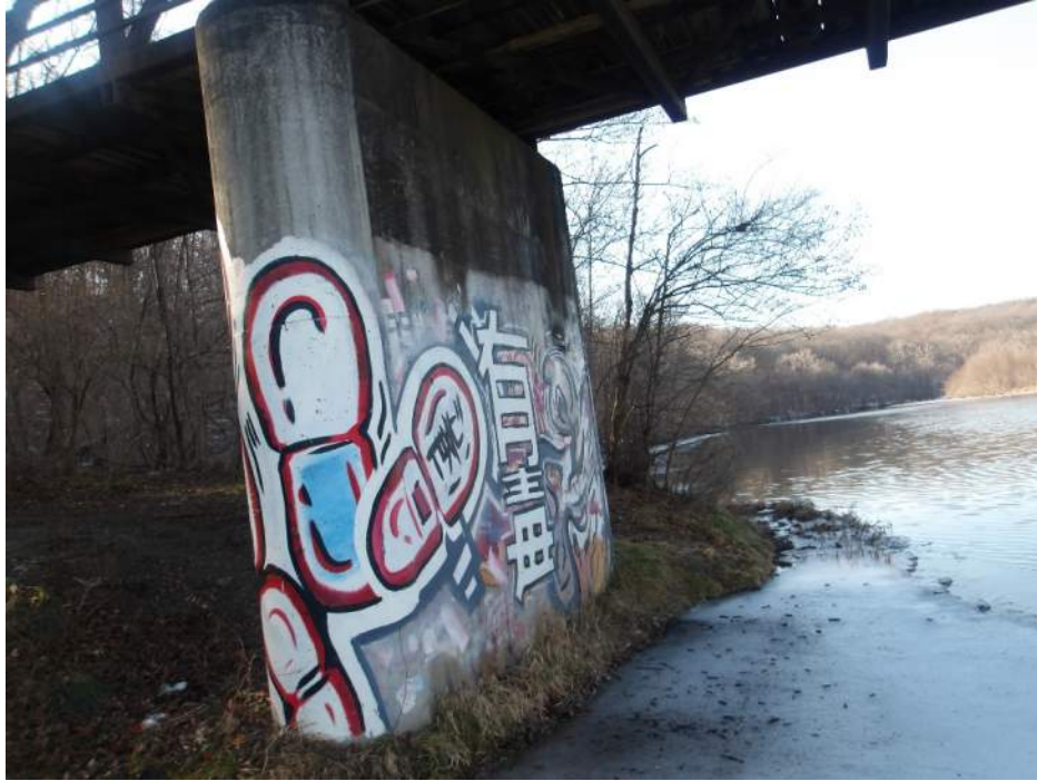
Photo 27 – Pier 1S North Face (Looking Southwest)
