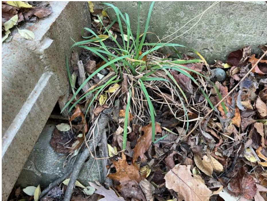
Photo 40 – Buried Southwest Bearing (Looking South)
