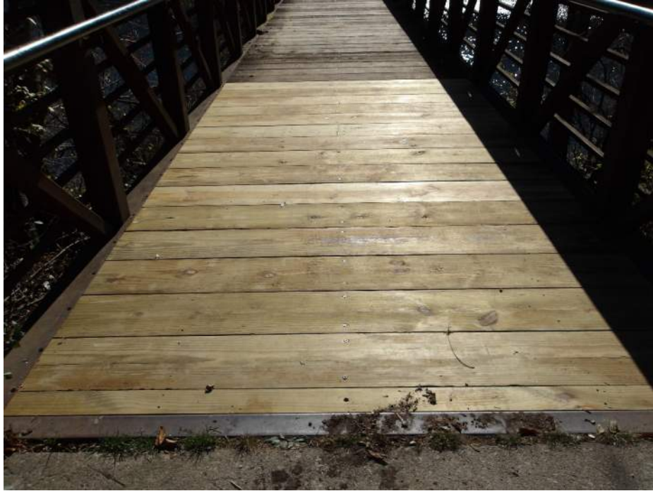
Photo 37 – Replaced Boards at North Abutment (Looking South)
