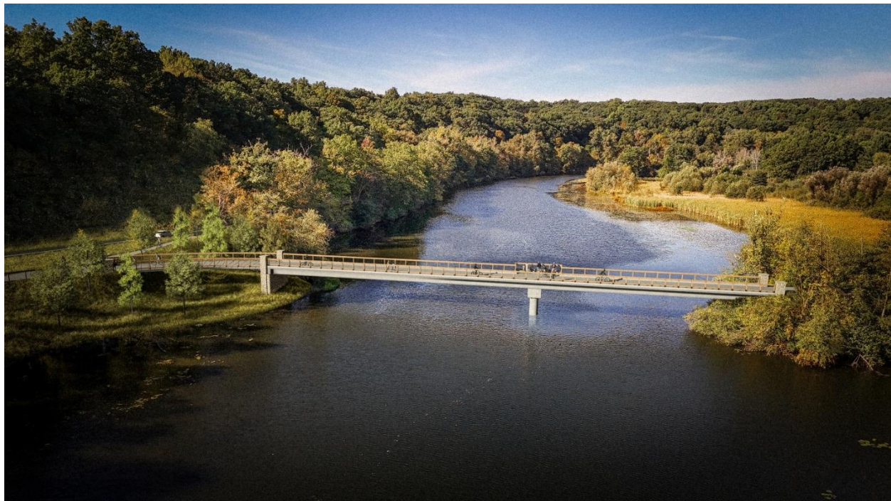
Figure 4 – Two-Span Steel Beam Bridge with Observation Platform
