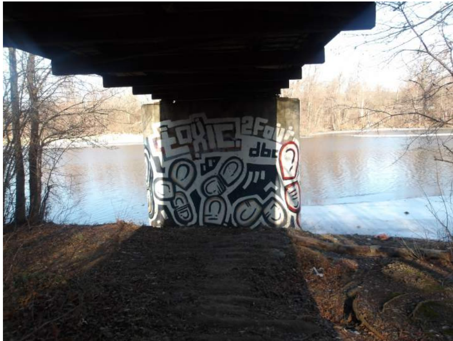
Photo 28 – Pier 1S South Face (Looking North)
