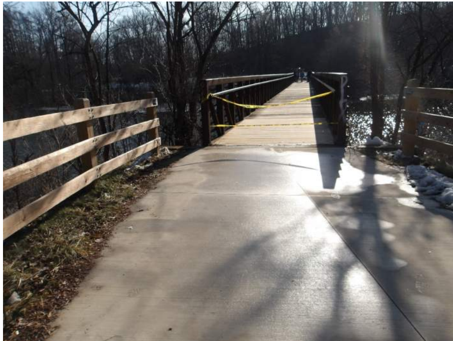
Photo 4 – North End of Structure (Looking South)
