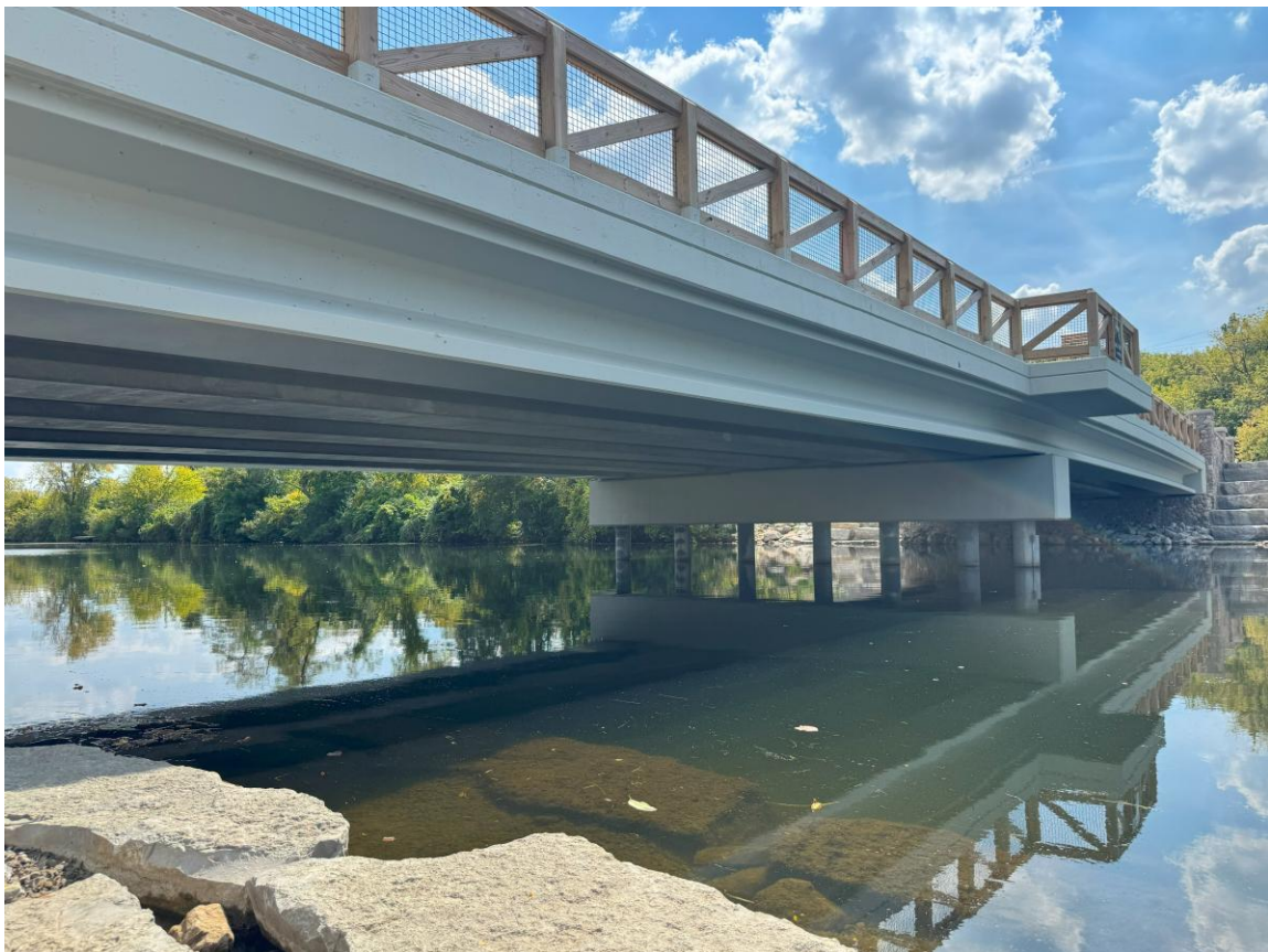
Figure 8 – Gallup Park Concrete Beam Bridge
