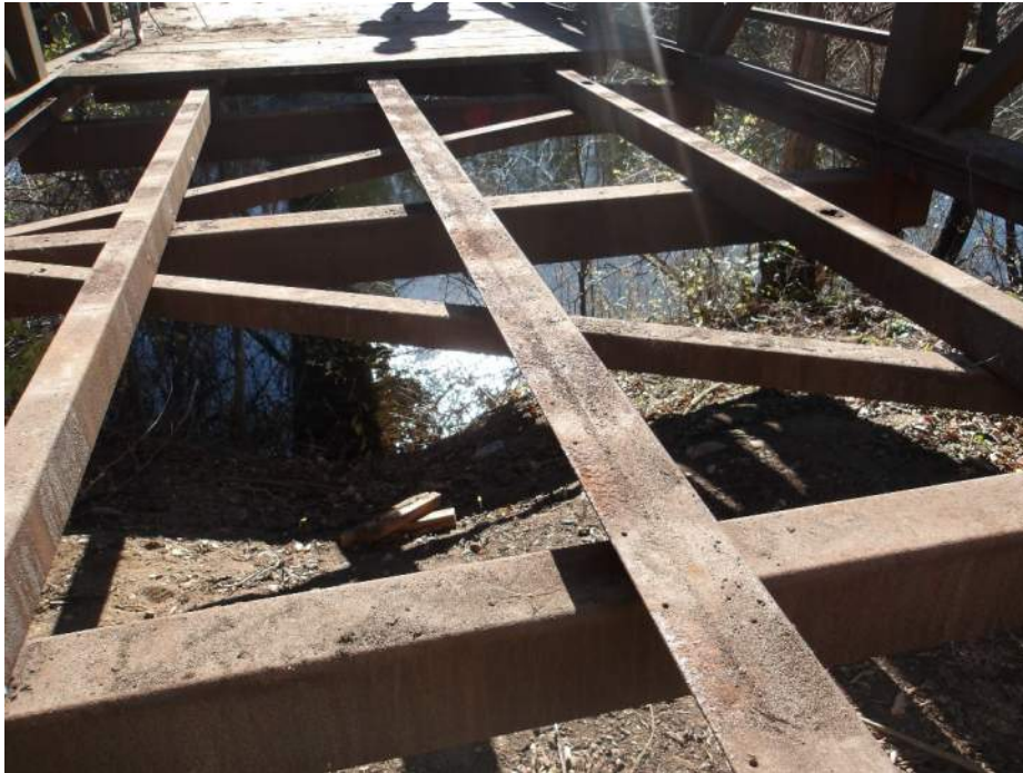
Photo 7 – Typical Beam 2W (Looking South)
