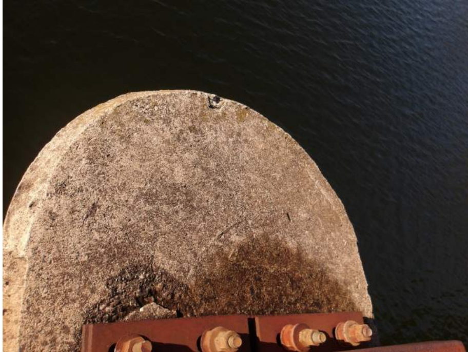
Photo 23 – Pier 2S West Pier Cap (Looking Northwest)
