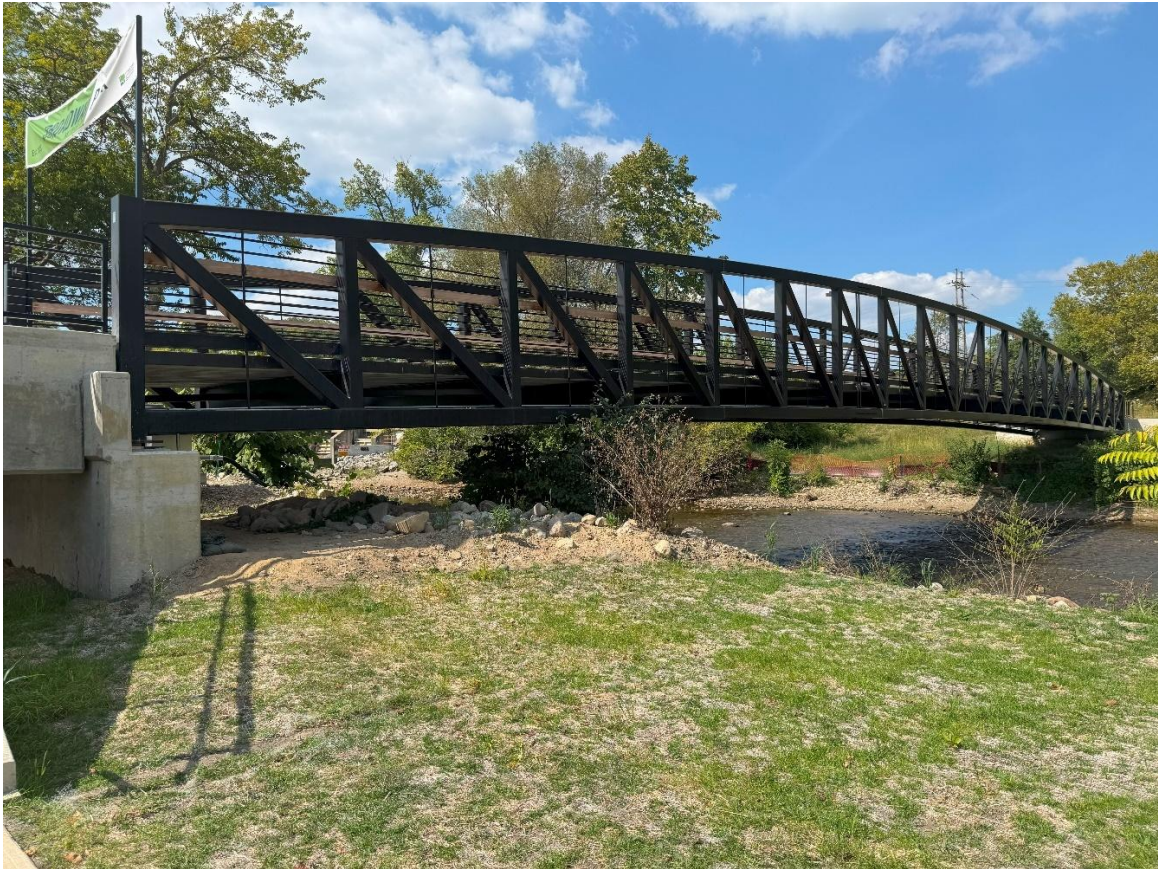
Figure 10 – Broadway Park Painted Steel Bridge
