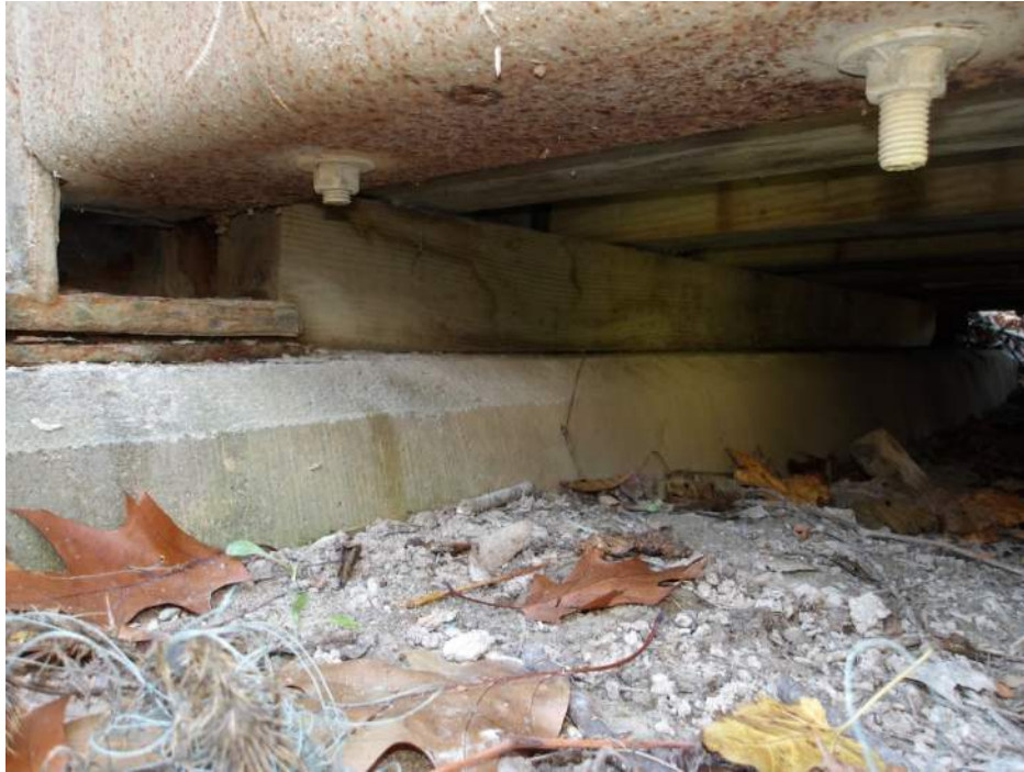
Photo 49 – South Abutment (Looking Southwest)
