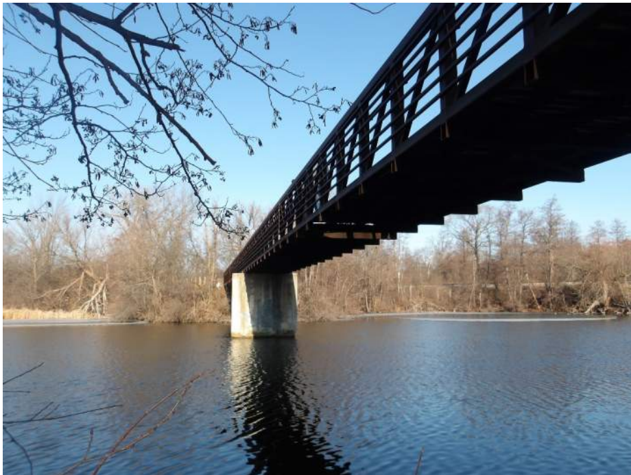
Photo 2 – West Elevation (Looking Northeast)
