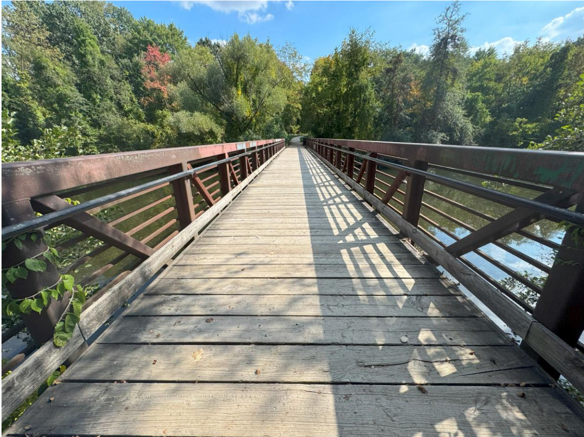
Figure 12 - North Barton Bridge Wooden Decking
