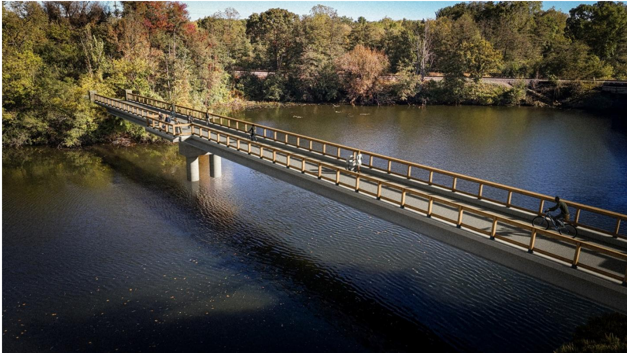
Figure 3 – Two-Span Steel Beam Bridge with Observation Platform
