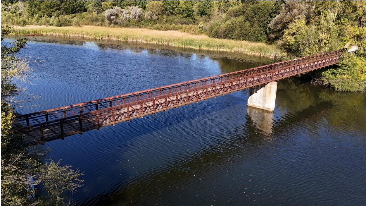
Figure 1 – Existing South Barton Bridge
