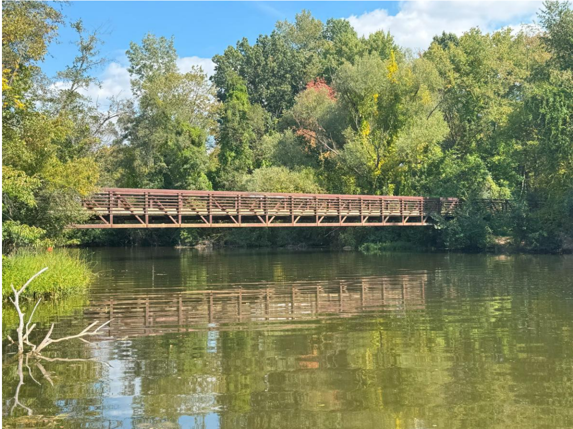
Figure 9 – North Barton Weathering Steel Bridge
