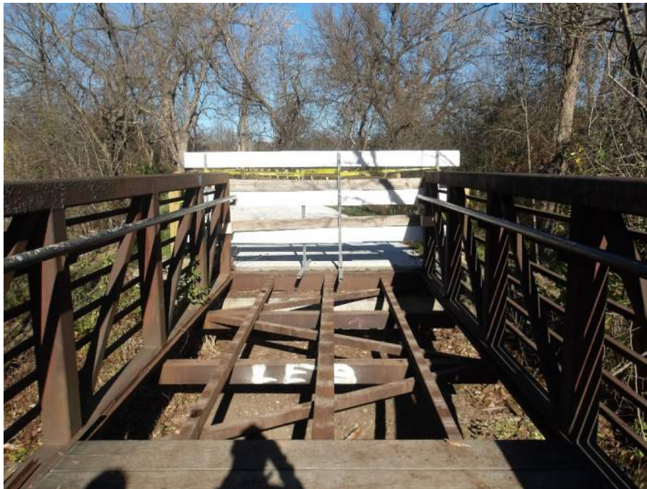
Photo 4 – Boards Removed for Inspection at North End (Looking North)
