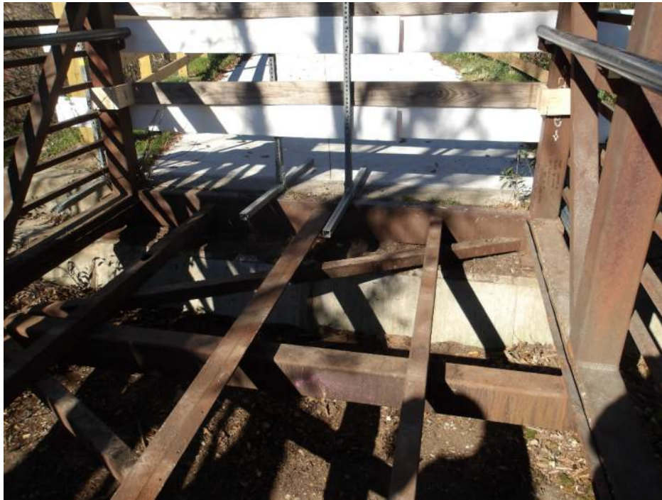
Photo 47 – North Abutment and tops of stringers (Looking North)
