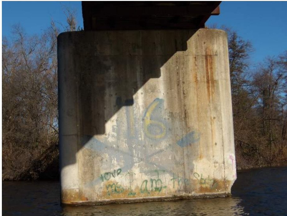
Photo 46 – Pier 2S south face (Looking North)
