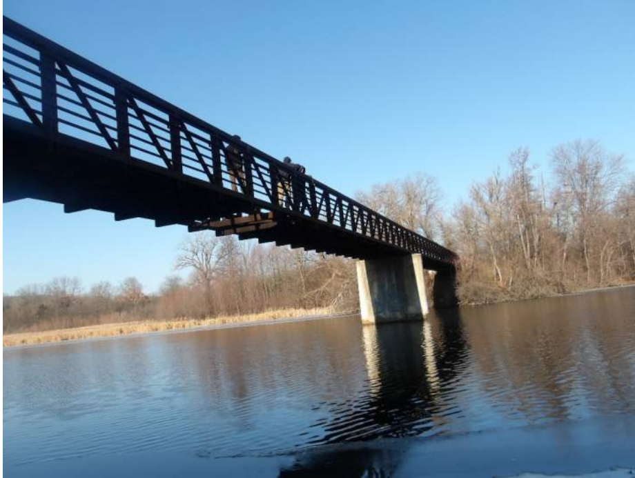
Photo 1 – East Elevation (Looking Northwest)
