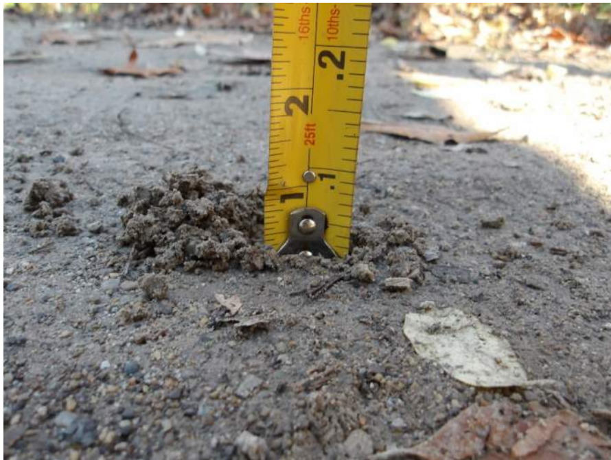
Photo 18 – 1/4" Deep Dirt and Debris (Looking East)
