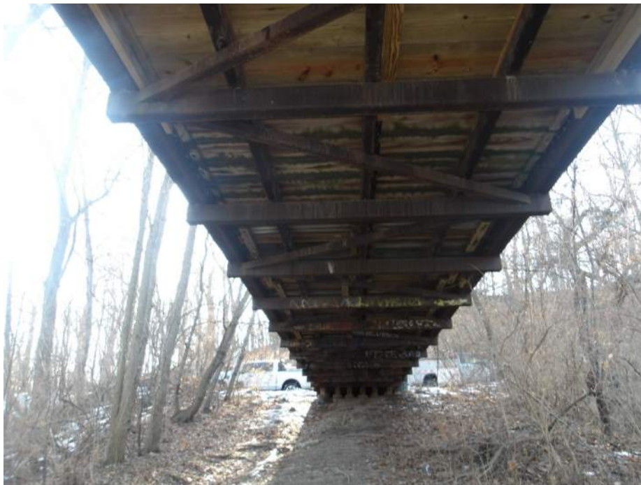
Photo 18 – Deck Underside Span 1 (Looking South)
