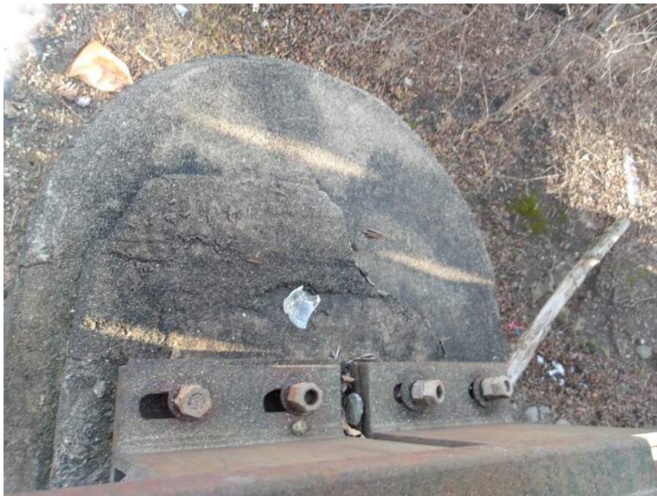
Photo 22 – Pier 1S East Pier Cap (Looking Southeast)
