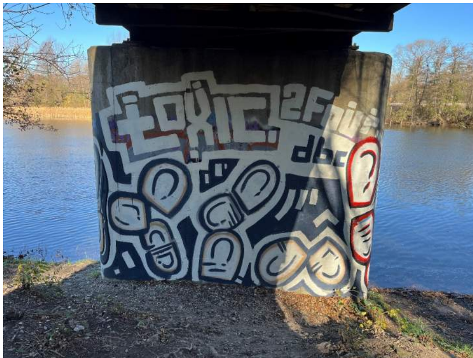
Photo 44 – Pier 1S south face (Looking North)
