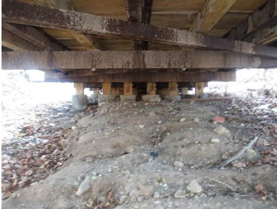
Photo 17 – Deck Underside Span 1 (Looking South)
