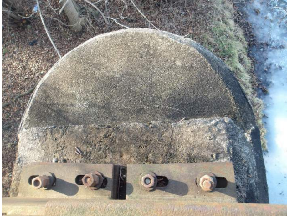
Photo 21 – Pier 1S West Pier Cap (Looking West)
