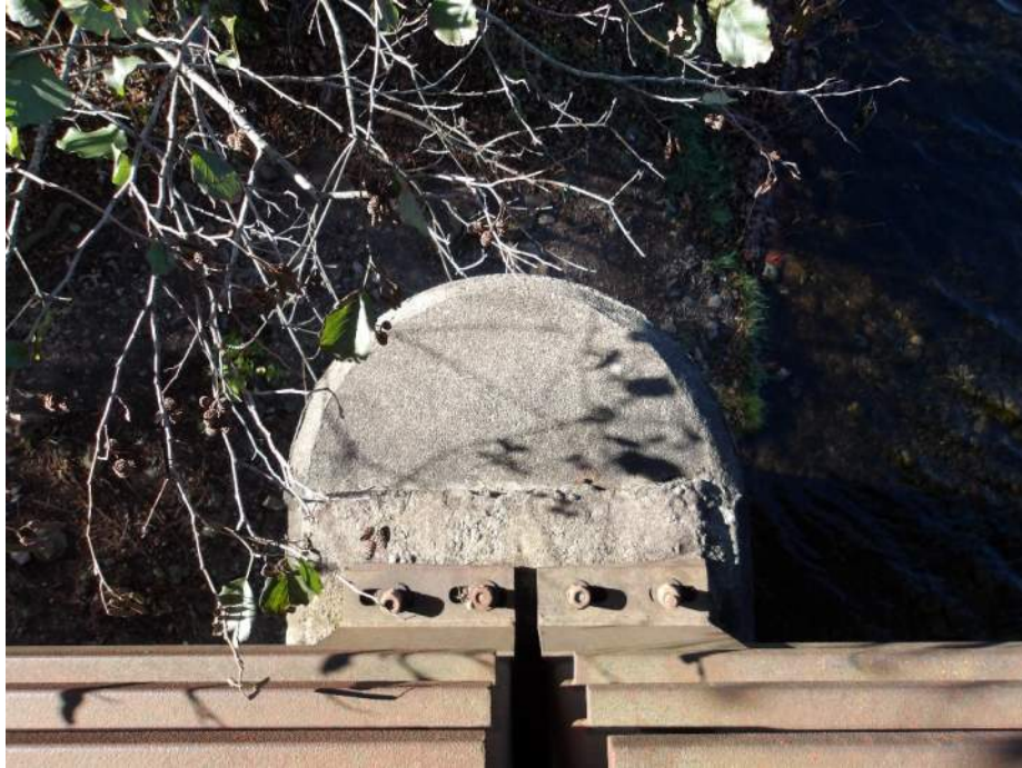
Photo 33 – Pier 1S West Pier Cap (Looking West)
