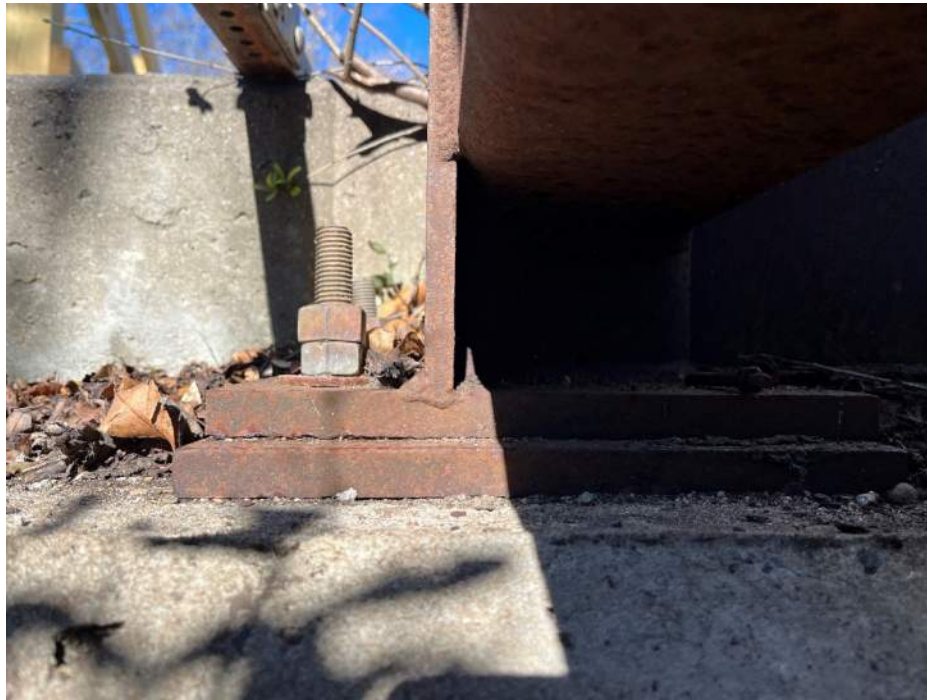
Photo 41 – Northwest Bearing (Looking North)
