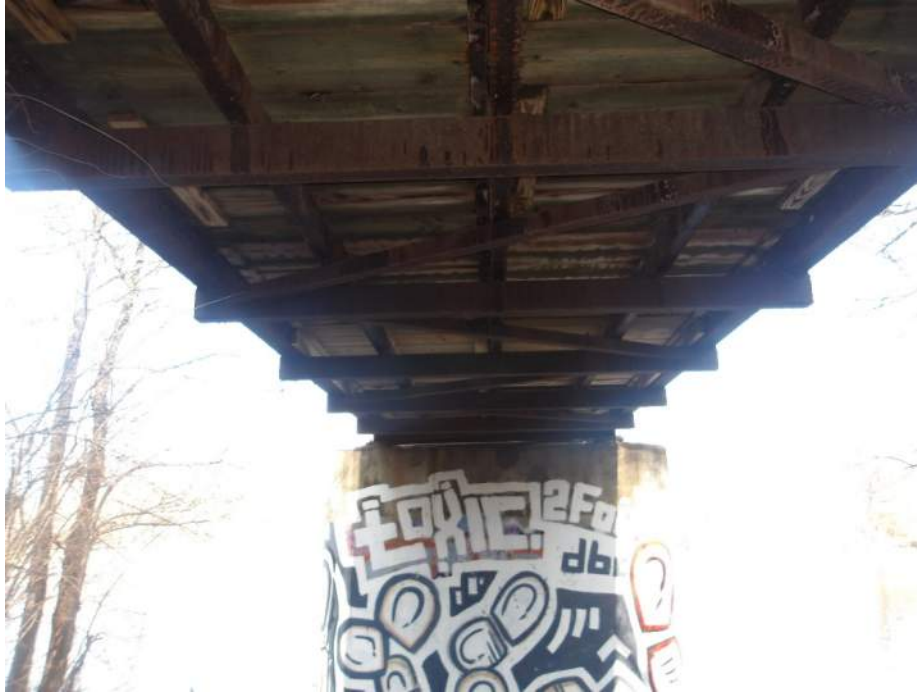
Photo 19 – Deck Underside Span 1 (Looking North)
