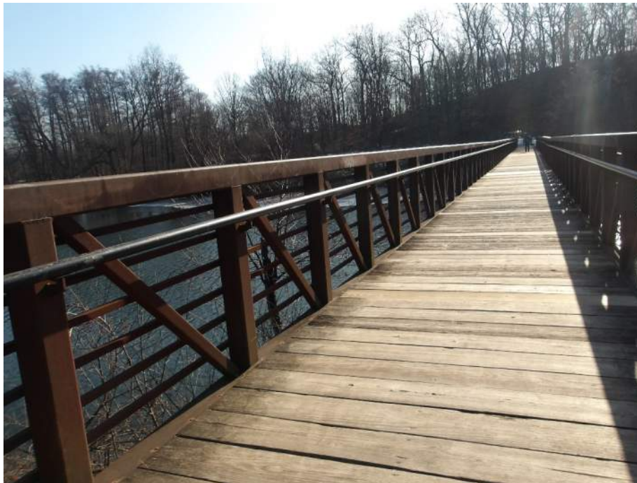
Photo 12 – Typical Condition of East Railing (Looking Southeast)
