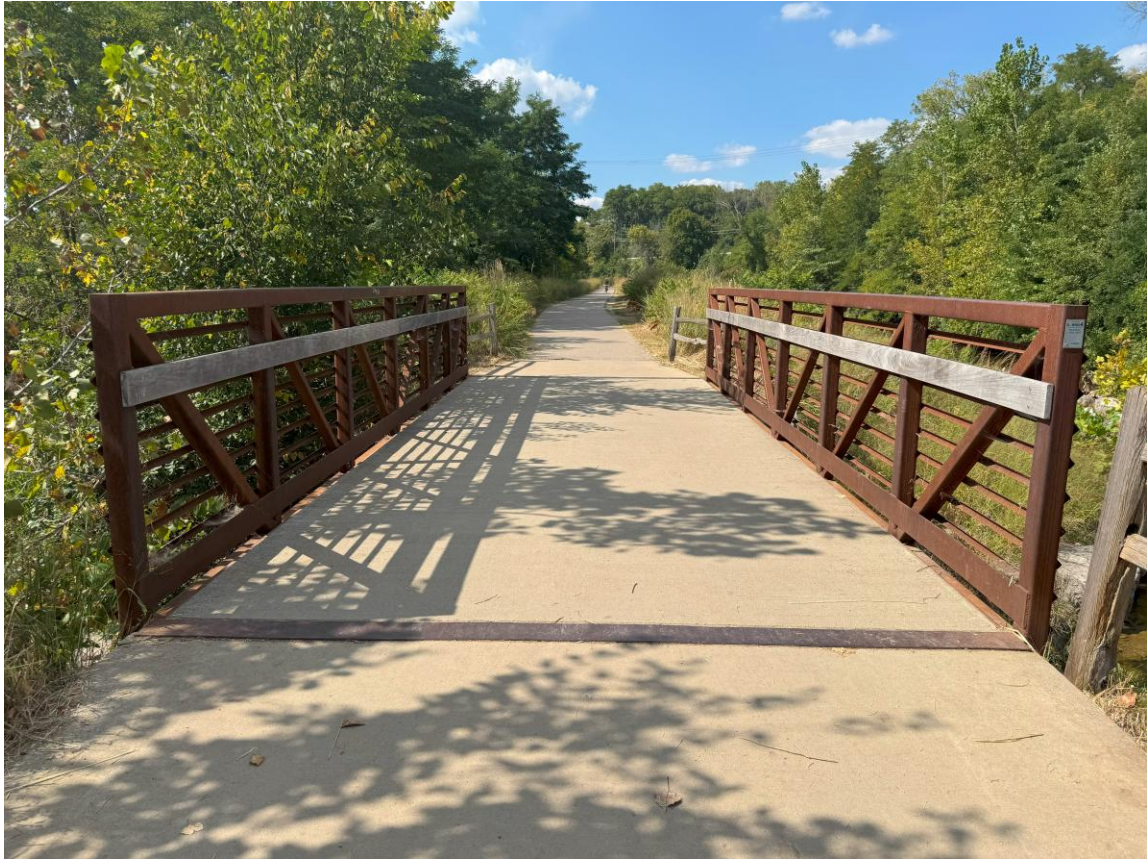
Figure 13 - Argo Park Bridge Concrete Decking
