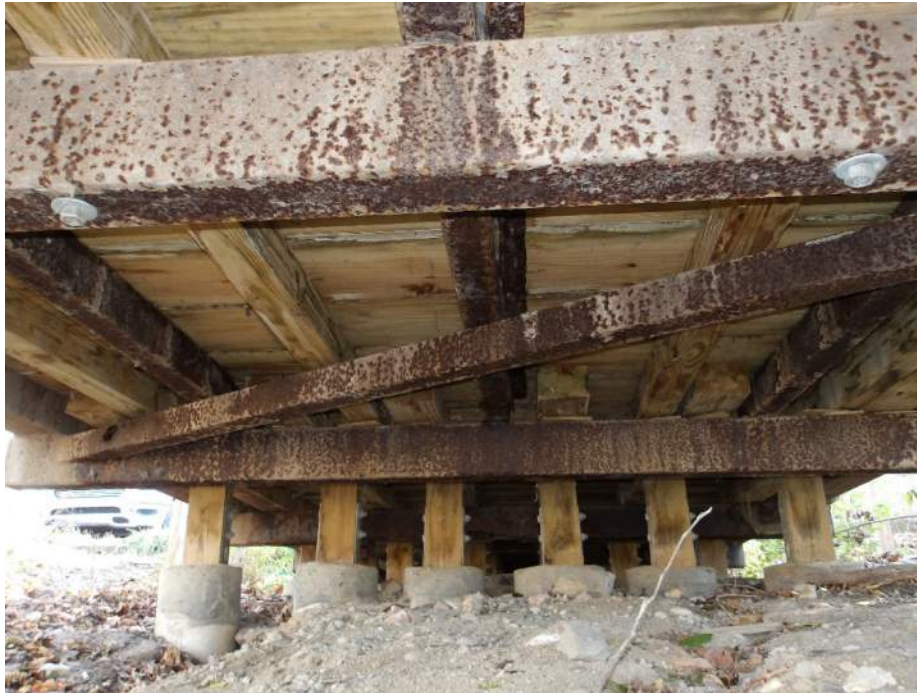
Photo 27 – Deck Underside between Floorbeams 4S and 5S (Looking South)
