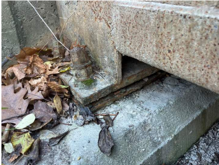
Photo 39 – Southeast Bearing (Looking Southwest)
