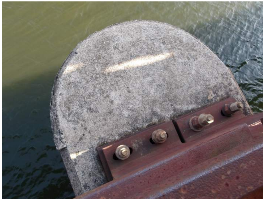
Photo 24 – Pier 2S East Pier Cap (Looking Southeast)
