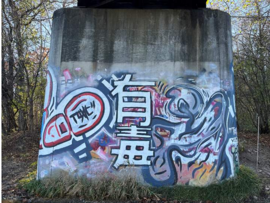
Photo 29 – Elevation Pier 1S North Face (Looking South)
