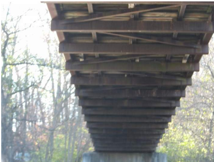
Photo 28 – Span 2 Underside from Pier 2S (Looking South)
