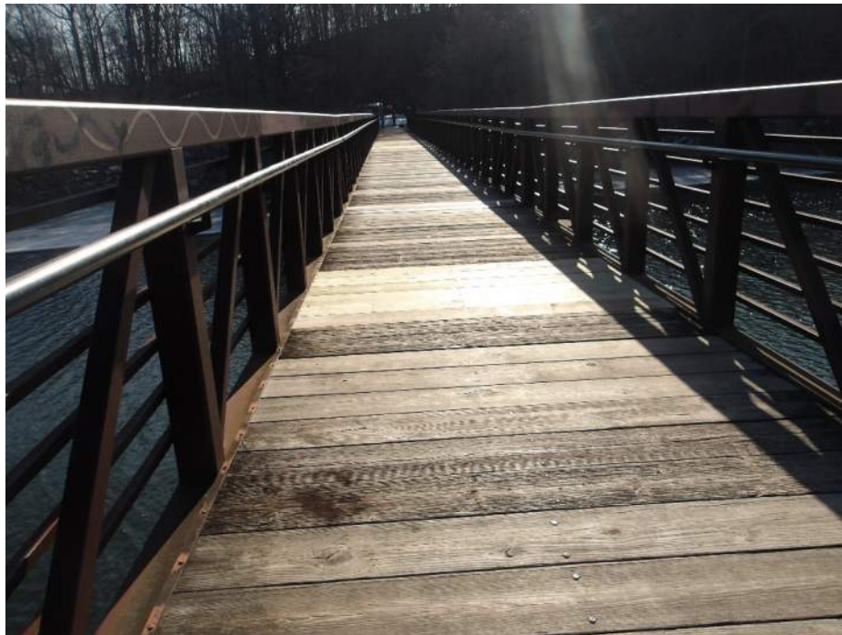
Photo 10 – Typical Deck with New Boards Placed (Looking South)
