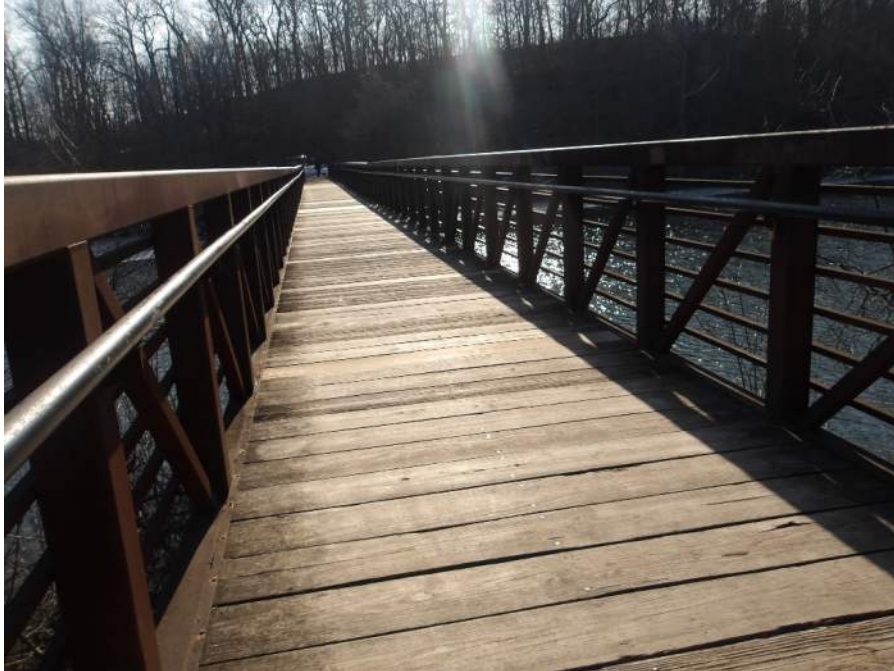
Photo 13 – Typical Condition of West Railing (Looking Southwest)
