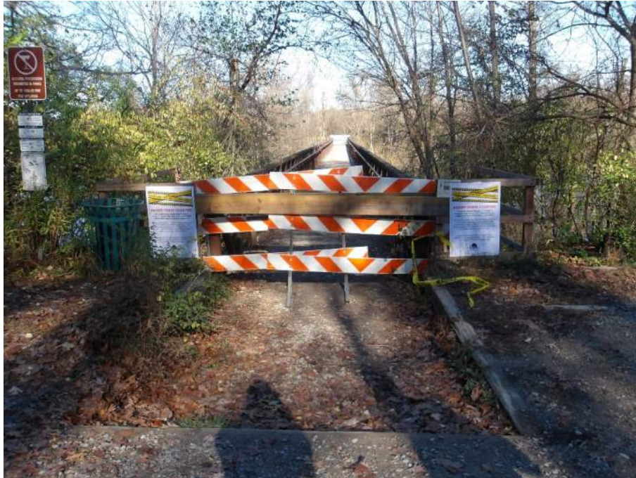
Photo 3 – South End of Structure (Looking North)
