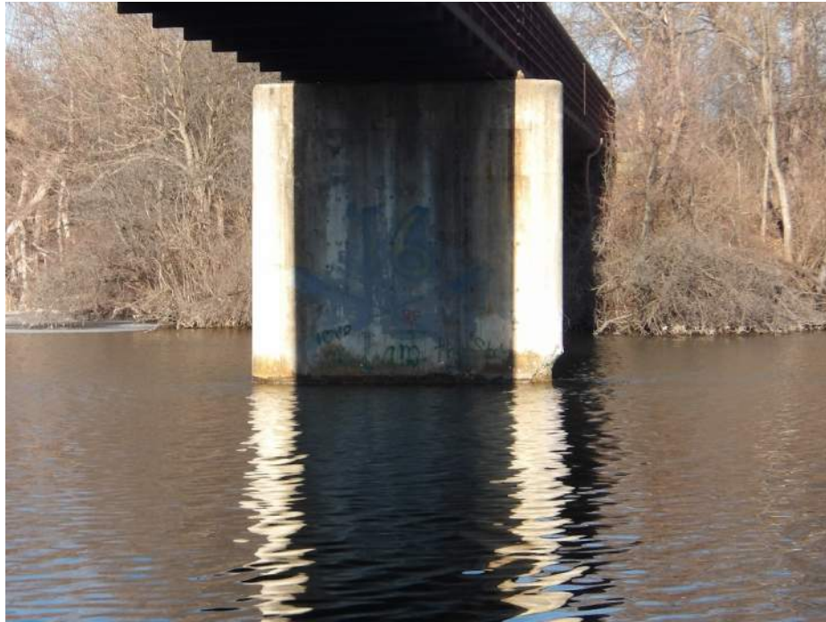
Photo 29 – Pier 2S South Face (Looking North)
