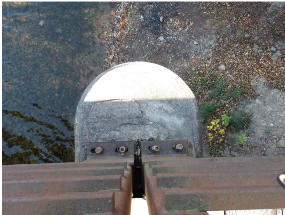
Photo 34 – Pier 1S East Pier Cap (Looking East)
