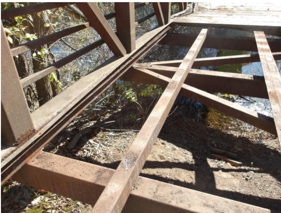
Photo 8 – Typical Beam 3W (Looking South)
