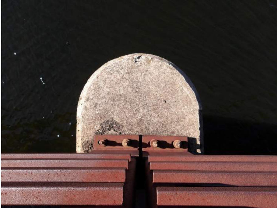
Photo 35 – Pier 2S West Pier Cap (Looking West)
