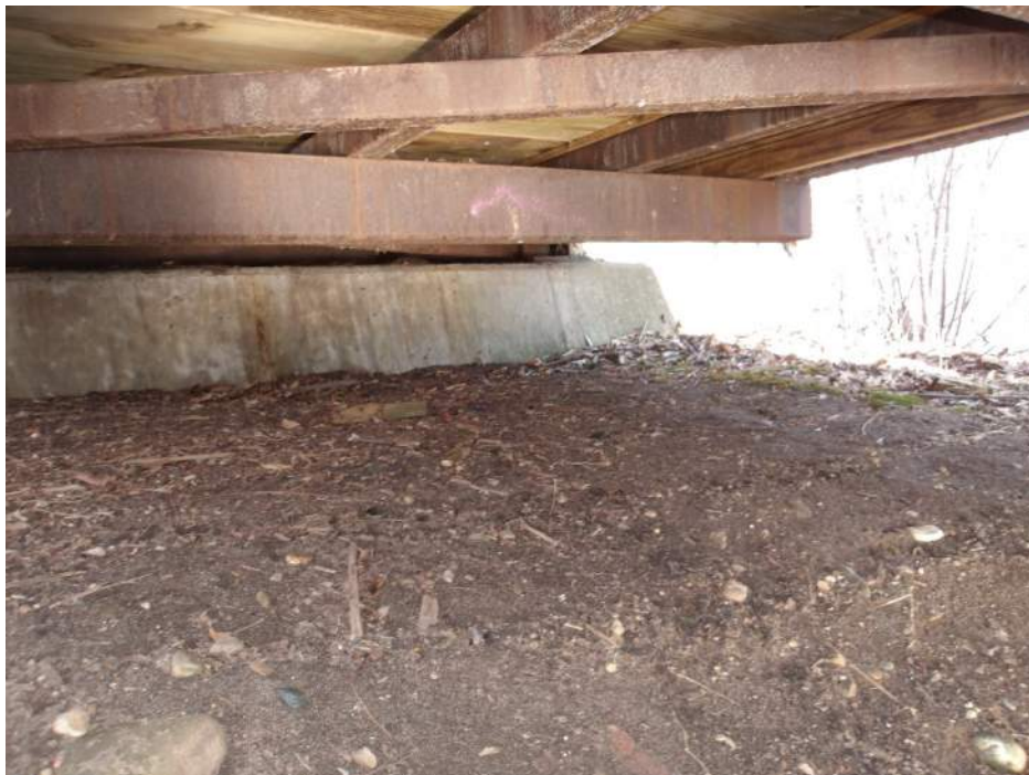
Photo 32 – North Abutment (Looking Northeast)
