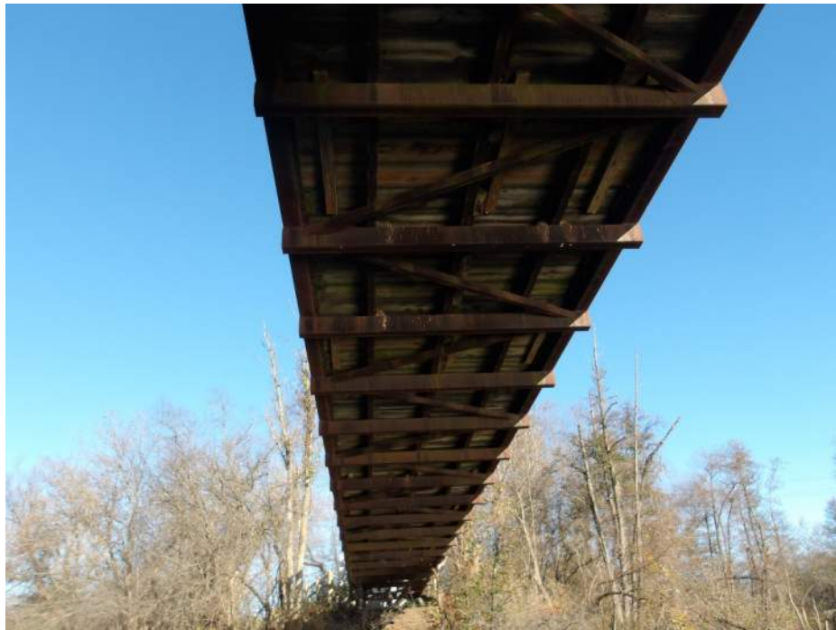
Photo 50 – Deck underside Span 3 (Looking North)
