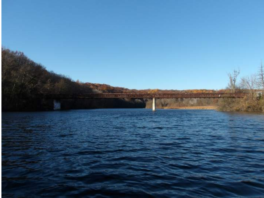
Photo 1 – East Elevation (Looking West)
