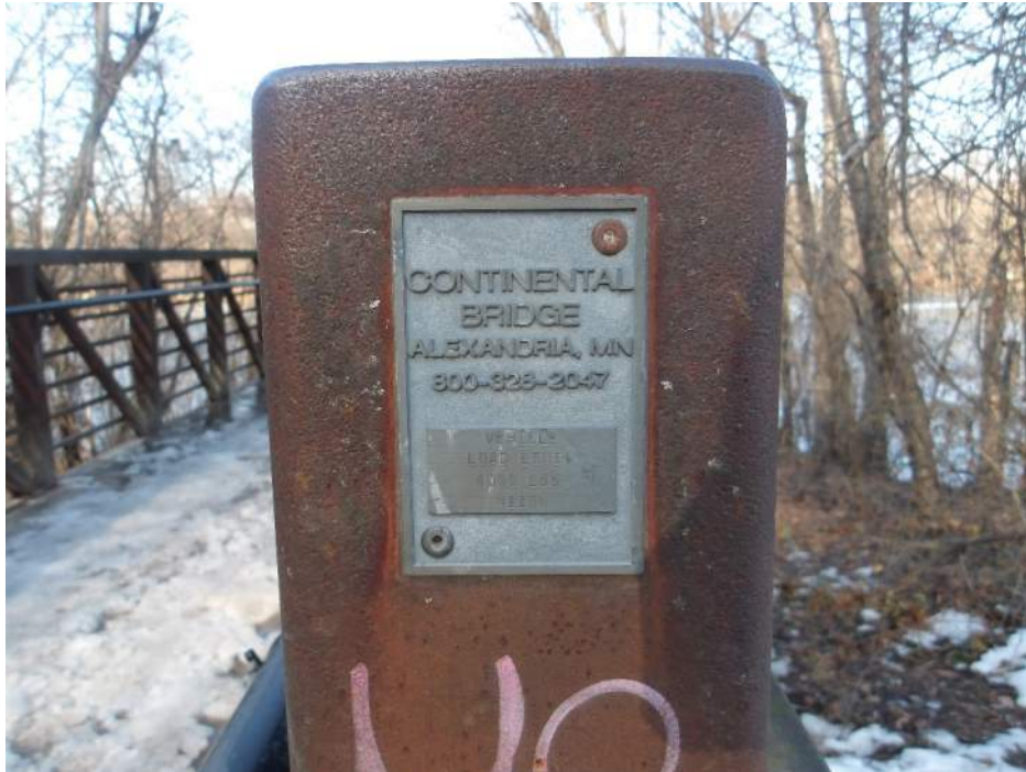
Photo 25 – Structure Nameplate (Looking North)
