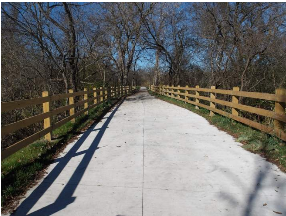
Photo 2 – North End Approach (Looking North)
