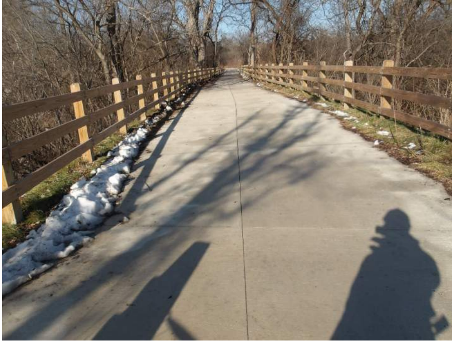
Photo 3 – North End Approach (Looking North)
