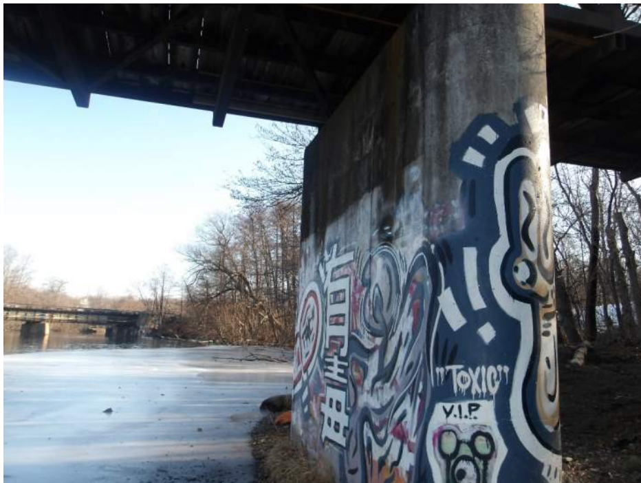
Photo 26 – Pier 1S North Face (Looking Southeast)
