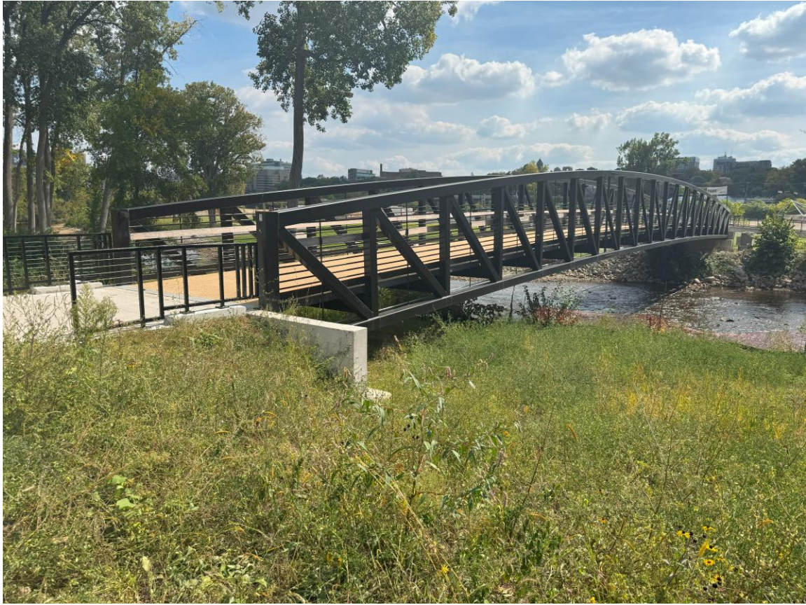
Figure 7 – Broadway Park West Prefabricated Bridge
