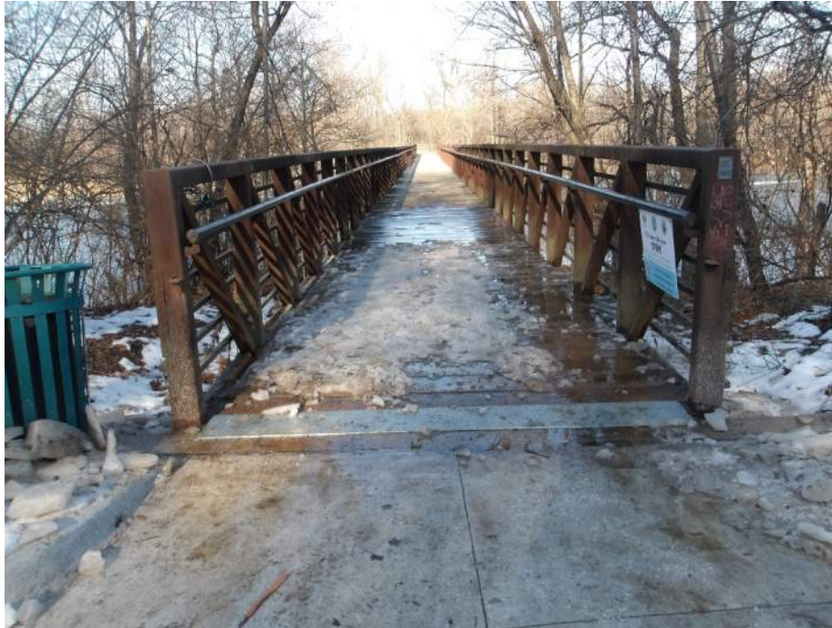
Photo 5 – South End of Structure (Looking North)
