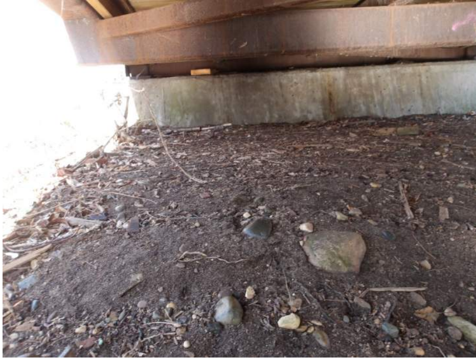
Photo 31 – North Abutment (Looking Northwest)
