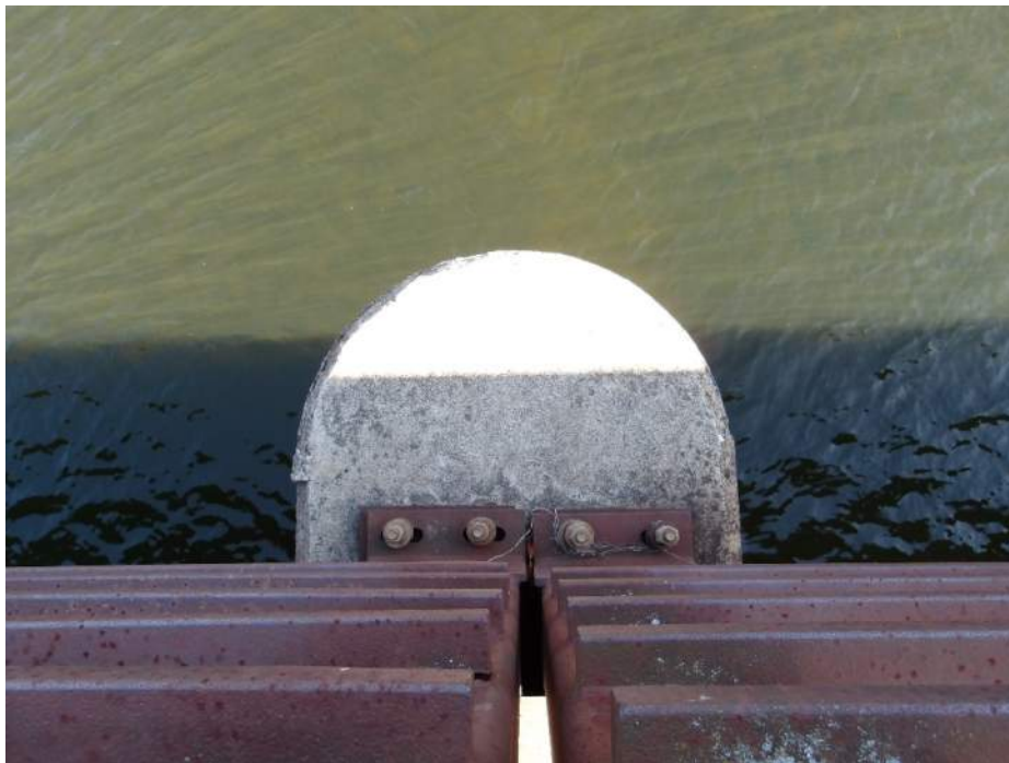
Photo 36 – Pier 2S East Pier Cap (Looking East)
