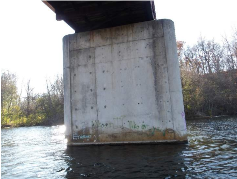
Photo 45 – Pier 2S north face (Looking South)
