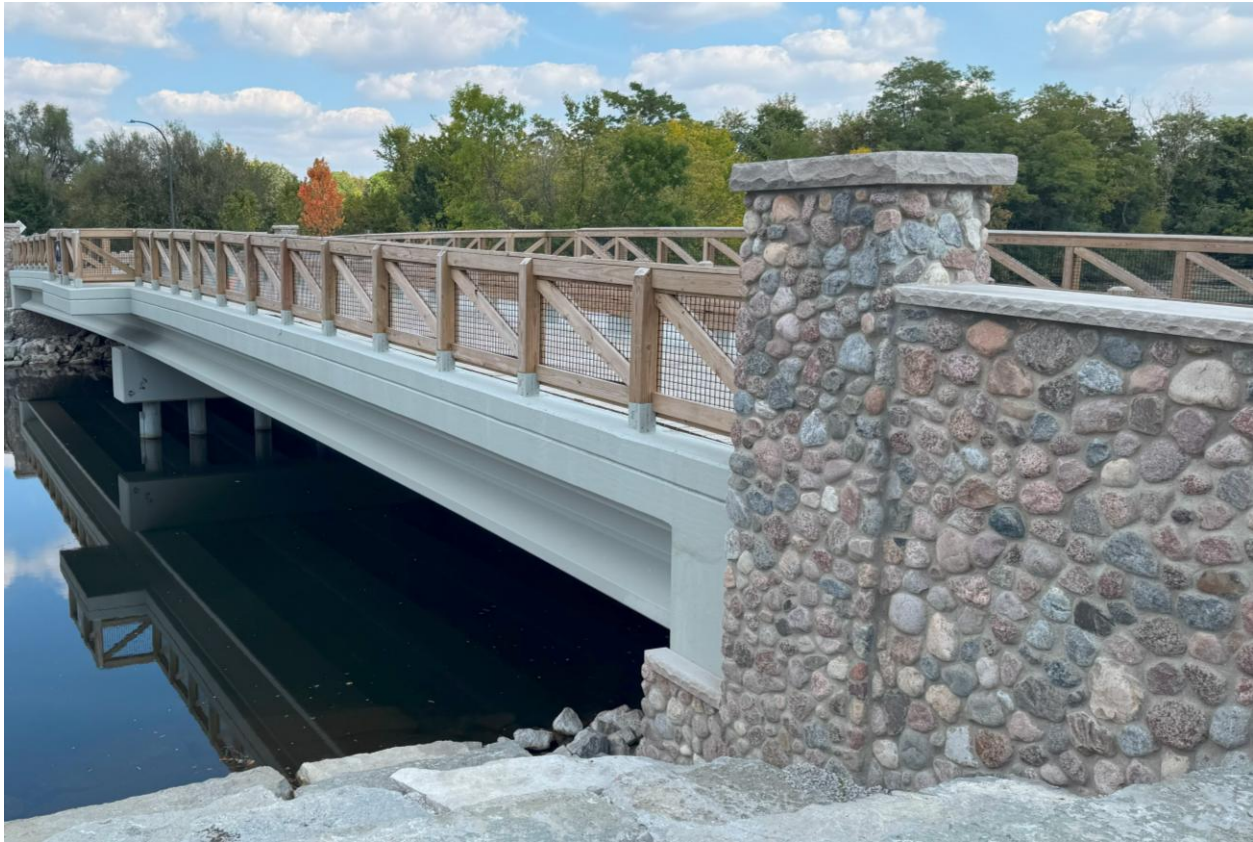
Figure 19 – Gallup Park Entrance Column and Railing
