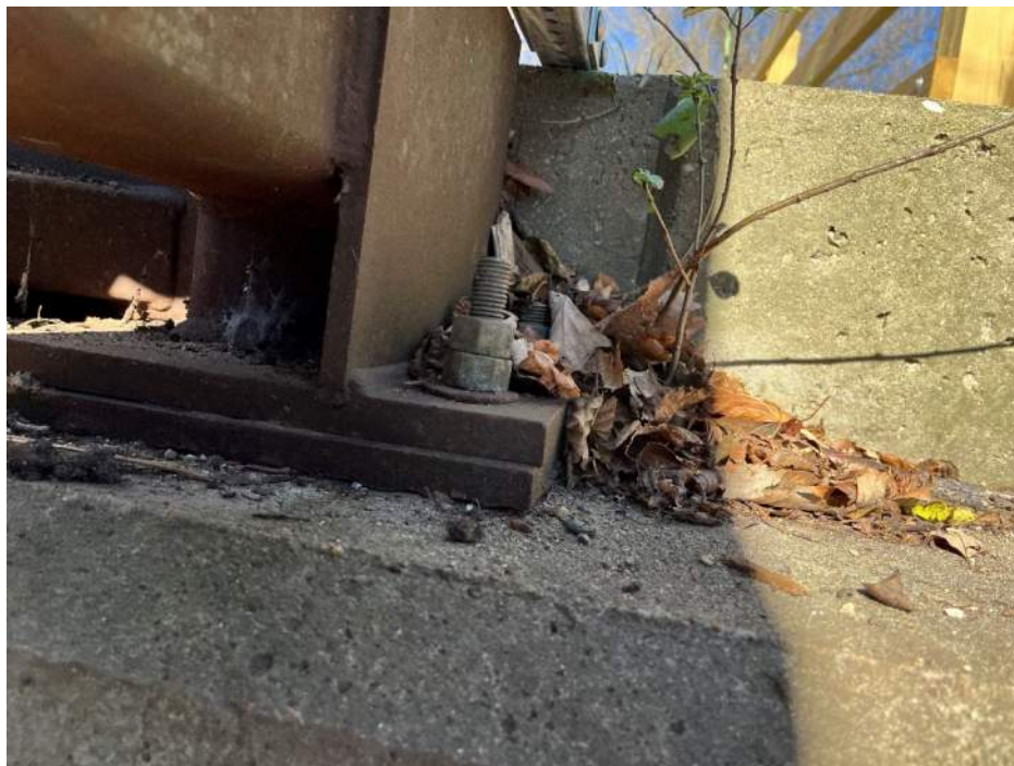
Photo 42 – Northeast Bearing (Looking North)
