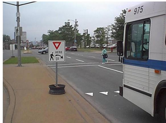
**Fig. 2.4W. Unsignalized Mid-block Crosswalk With Parking Guidelines**
