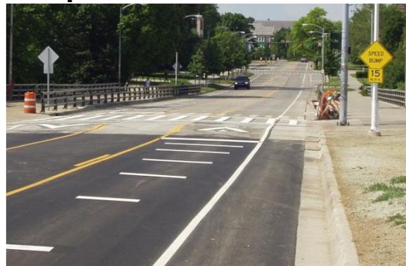
**Fig. 2.4Y. Mid-block Crosswalk with Crossing island Guidelines**
