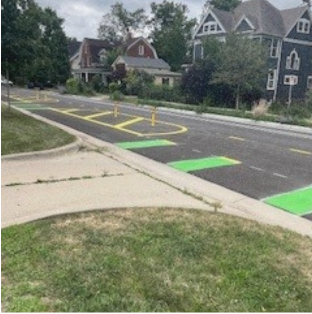
Fifth Ave. - Resurfacing
