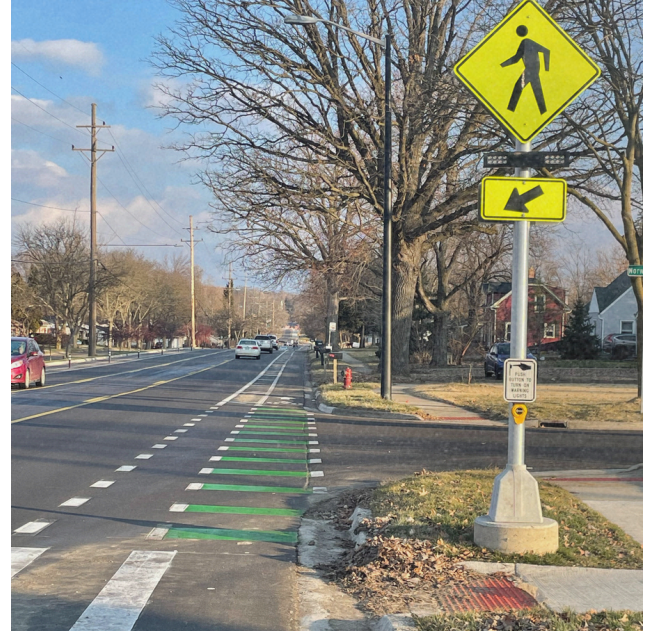
Platt Rd. - Resurfacing
