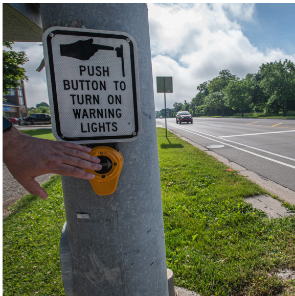
Accessible Pedestrian Signal
