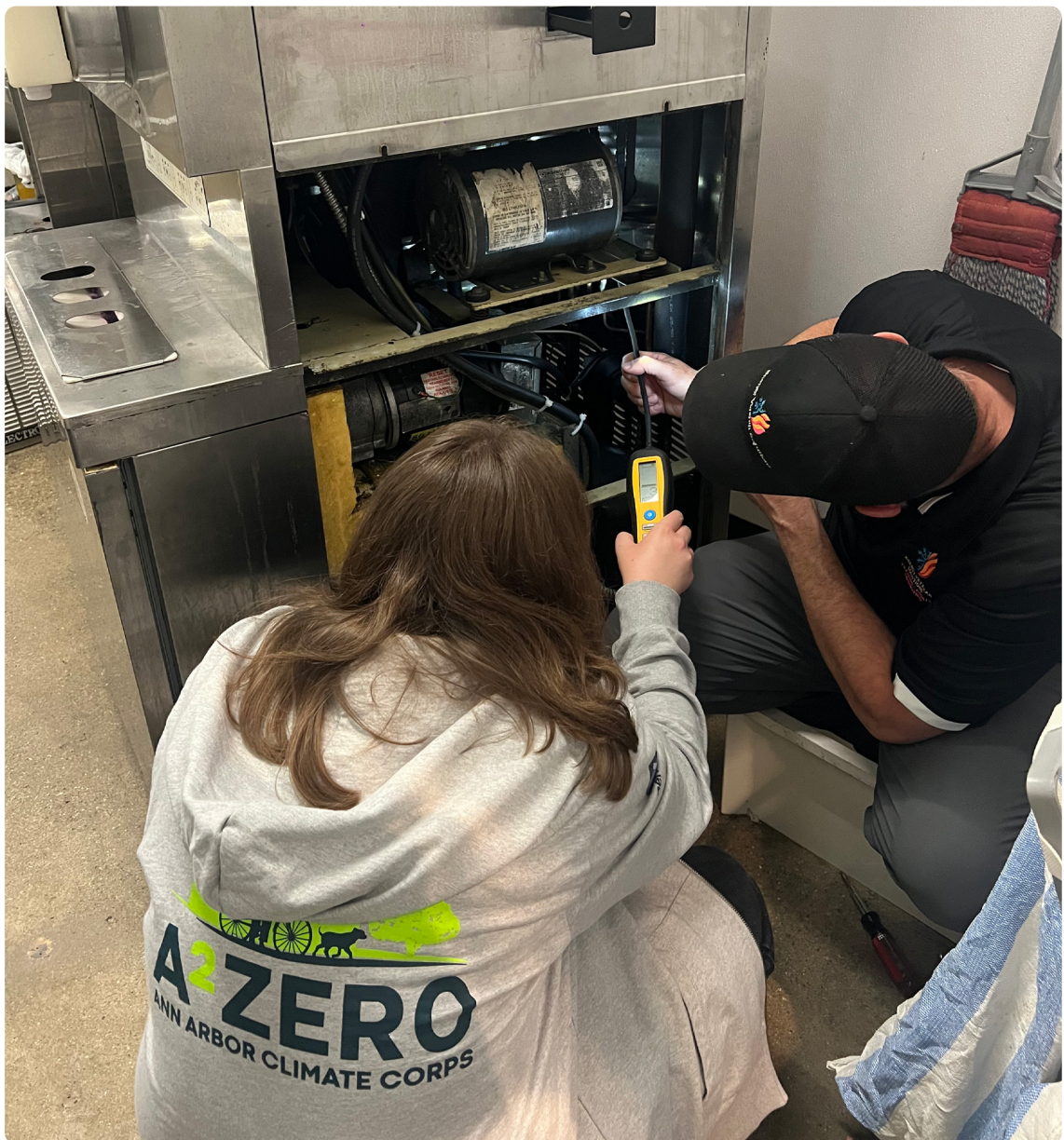
A refrigerant leak test at Bløm Meadworks.
