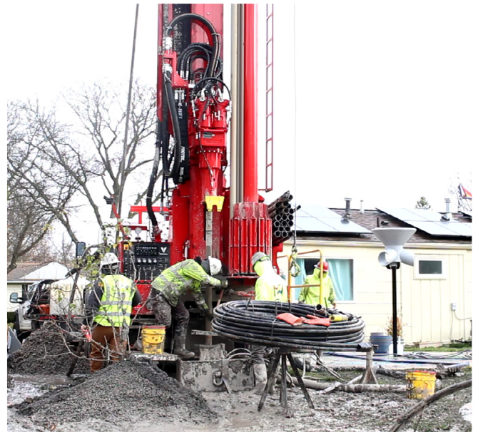
Drilling for the geothermal system at the Bryant Community Center.
