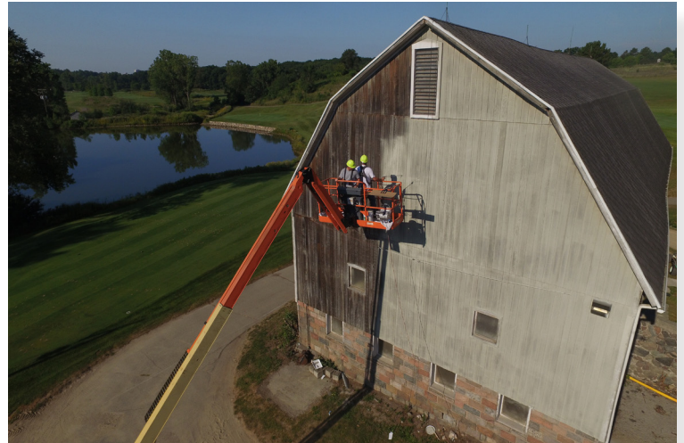
The maintenance barn being painted at Leslie Park Golf Course.
