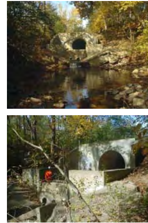
Figures 3.8 (a) and (b) Examples of Large Concrete Culverts in Millers Creek
