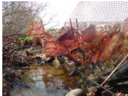
Figure 1.1 Damage on Pfizer Campus Along Millers Creek
