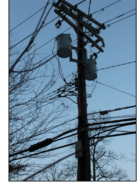
1 PHOTO POWER POLE SCALE: NA
