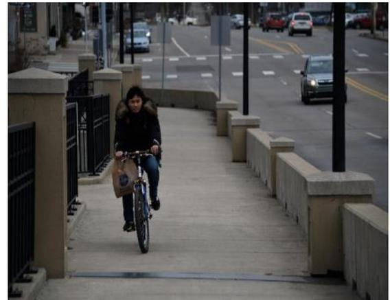
**Figure 5: Broadway Street bridge has poor visibility around the curve at Division Street and concrete pillars holding light poles extend too far into the travel way. Concrete fillers should be placed to eliminate the protrusions of the bridge and lighting posts, presenting a smooth barrier face to cyclists.**
