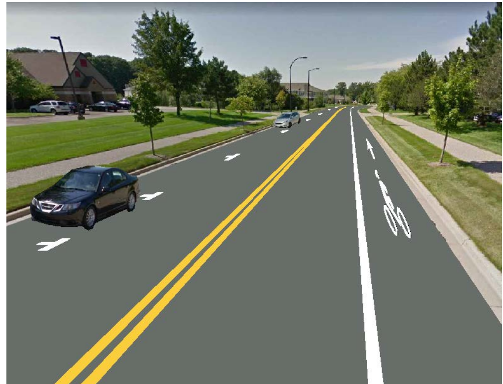
Potential (3 to 2) Lane Reconfiguration
