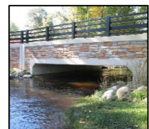
Figure 4: Three-sided box bridge
