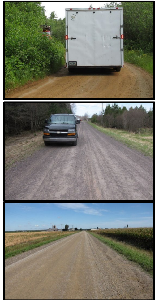
Figure 2: Top — Road with IBR number of 1 road that has poor surface width, poor drainage adequacy, and poor structural adequacy. Middle — Road IBR number of 7 that has fair surface width, fair drainage adequacy, and fair structural adequacy. Bottom — Road with IBR number of 9 road that has good surface width, good drainage adequacy, and good structural adequacy.
