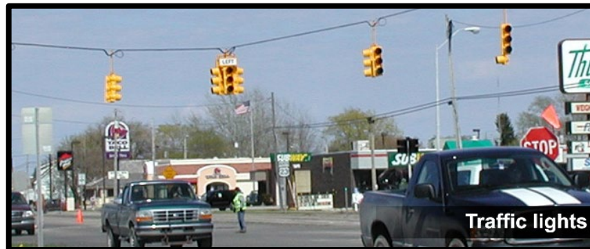
Figure D-1: Example of traffic signals
