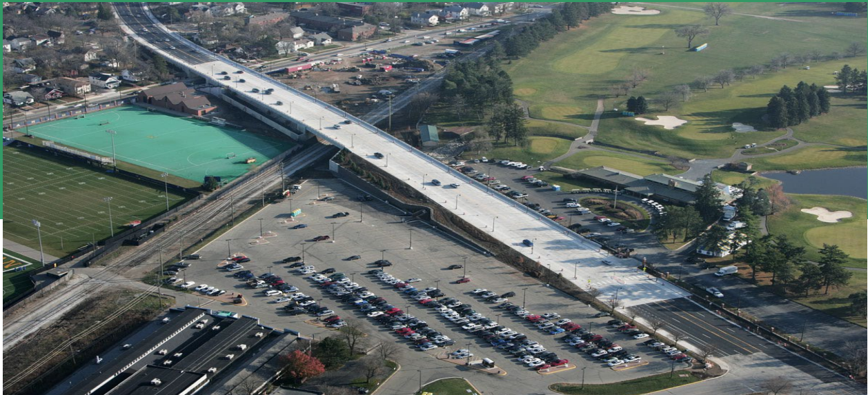
E. Stadium Boulevard Bridges – November 2012
