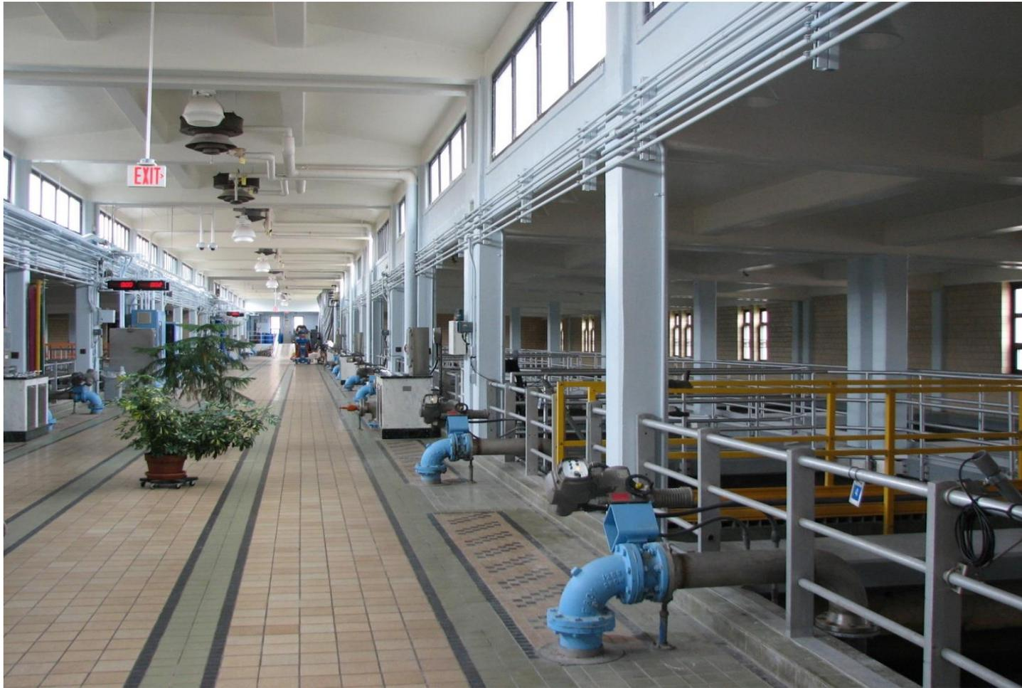
**Water Treatment Plant Filter Rehabilitation:** This project would modify the City’s existing filters to increase the depth of filter media. Increasing filter media depth will improve the City’s ability to remove certain emerging contaminants in its watershed, such as PFAS. This project will improve the quality of the City’s drinking water and reduce a known public health risk.
