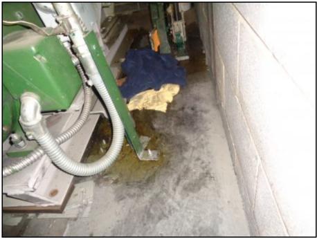
21 : View of elevator equipment leakage and staining
