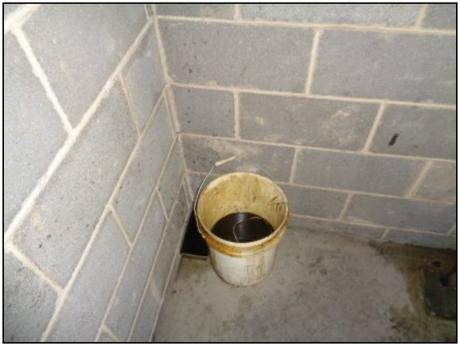
23 : View of elevator equipment leakage
