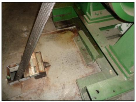
22: View of elevator equipment leakage and staining
