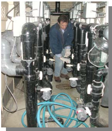
Figure 7. Sample Collection at the Wastewater Plant.
