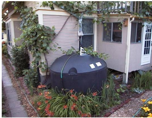
1500 gallon cistern fed from two gable downspouts. (Source: Experiments in Sustainable Urban Living )
