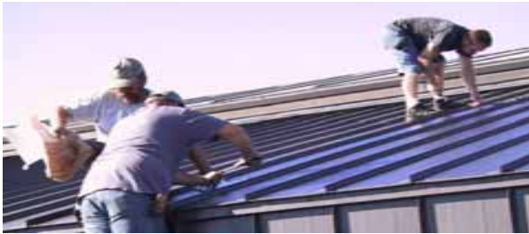
Installing solar on UM's Dana Building
