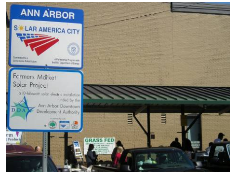
Farmers Market PV installation was completed in September 2008.
