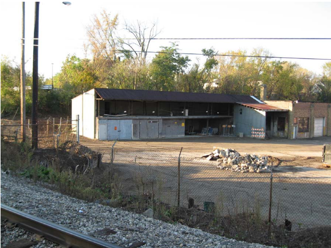
Figure 2 - View from east property line looking south
