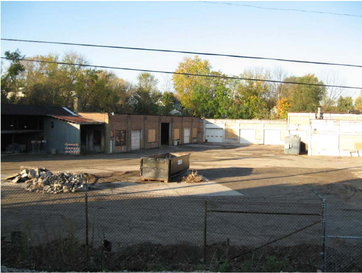
Figure 3 - View of buildings from east property line looking west
