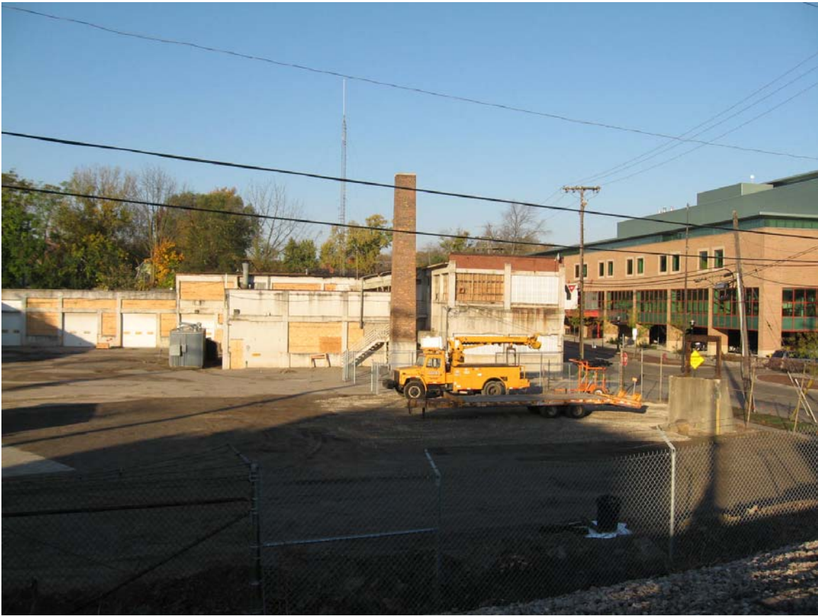
Figure 1 - View of building from east property line looking northwest
