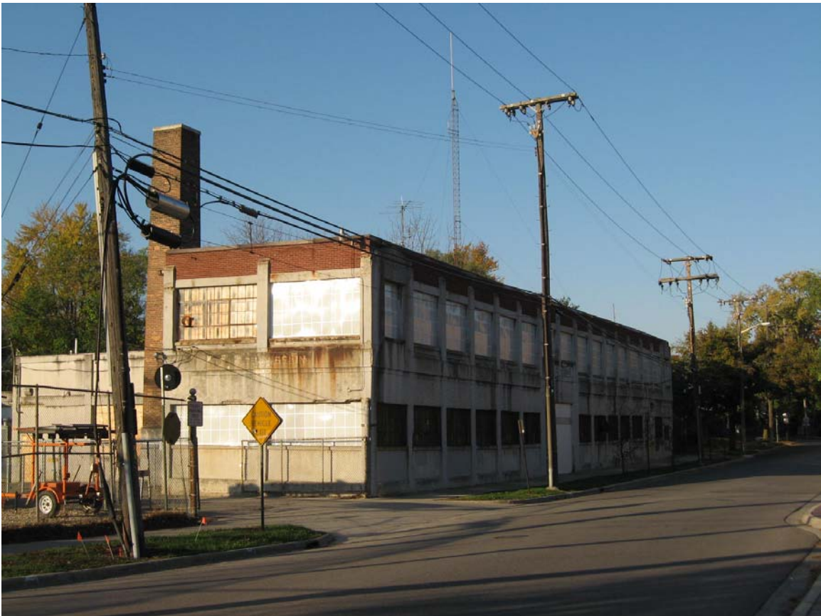
Figure 4 - View of main building from Washington Street, looking southwest
