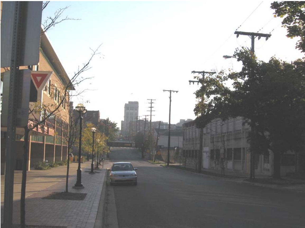
Figure 6 - Washington Street looking east to downtown
