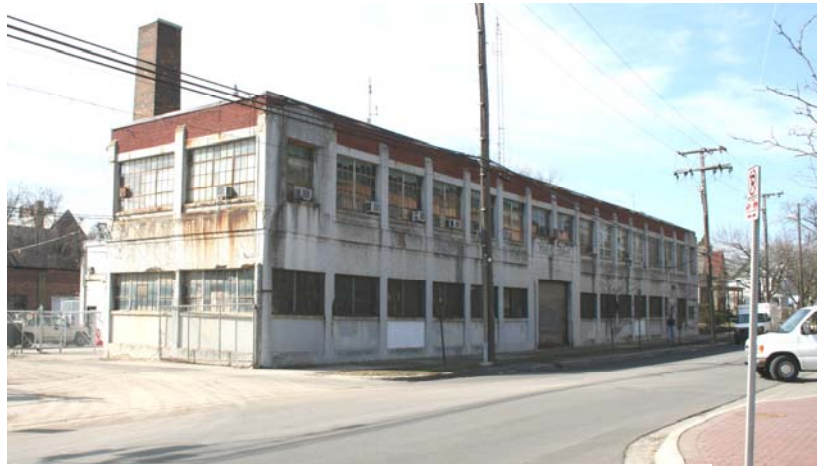
Fig 1. Main building façade along West Washington Street
