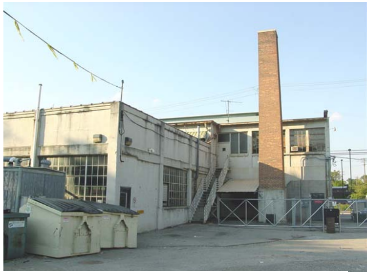
Fig 2. Main building, rear façade, looking north
