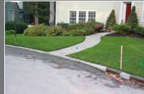
Harvard Place prior to construction
