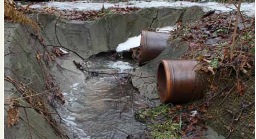
storm sewer outlet & channel prior to construction
