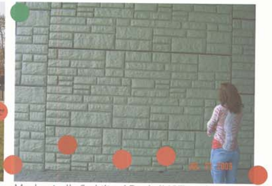
Mechanically Stabilized Earth (MSE) with Pre-cast Concrete Facing Panels
