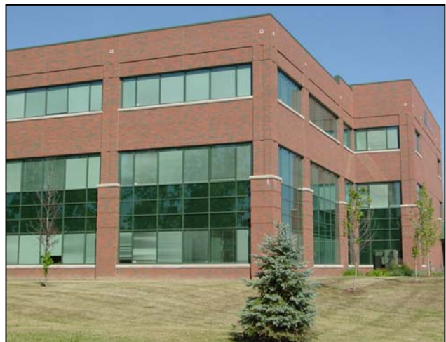
Multiple story office buildings can reduce imperviousness
