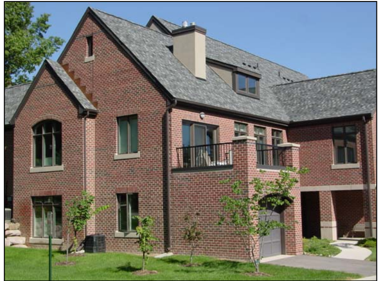
Private residential open space above a garage.
