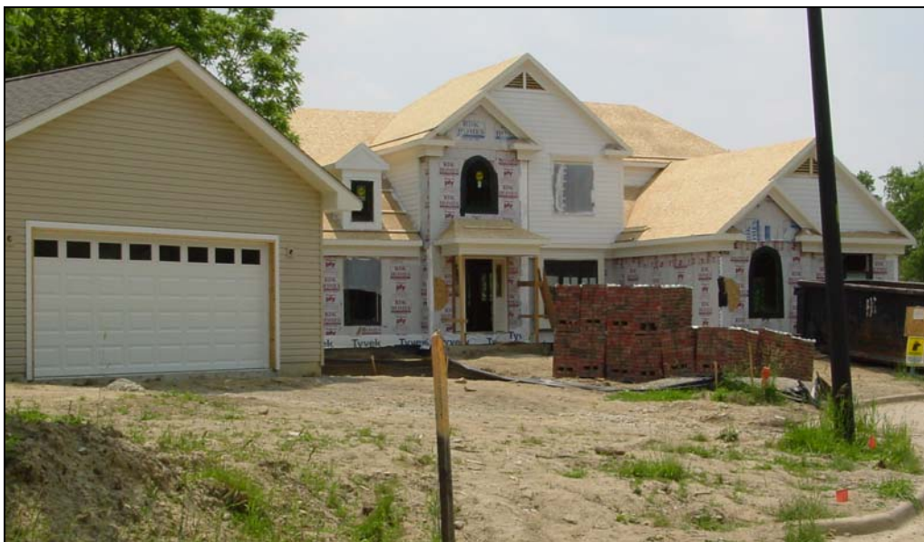
New Construction in the Northeast Area
