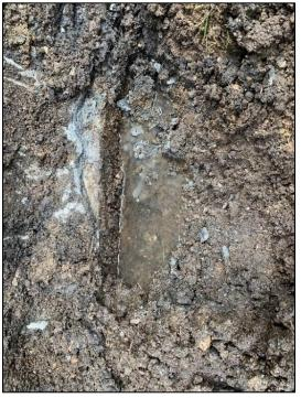
Photo 4: Saturated Top & Local Erosion Below Footing
