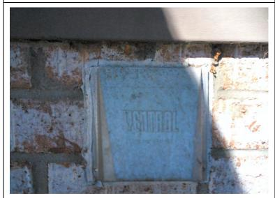
**Photo 5.** View of the asbestoscontaining dryer vent caulk
