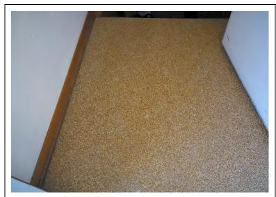
**Photo 4.** View of the asbestoscontaining linoleum in the entry area
