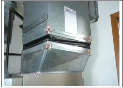
**Photo 6.** View of the presumed asbestos-containing vibration dampener
