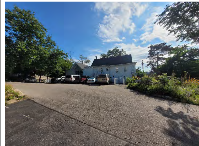
Photo 20. View of the east adjoining residential property
