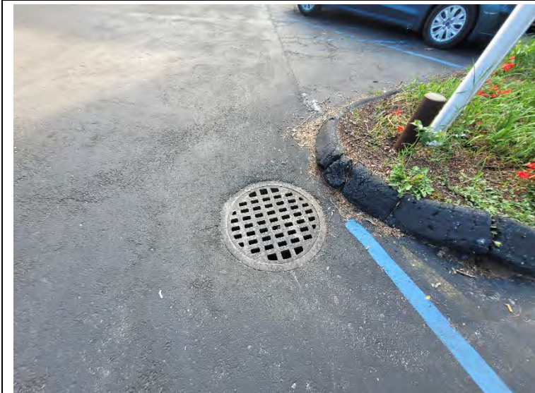
Photo 17. View of a storm water catch basin
