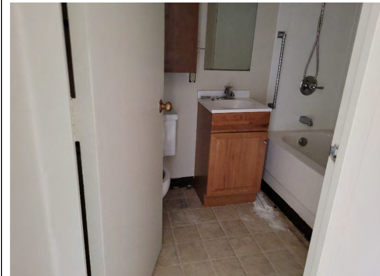
Photo 12. View of a typical bathroom
