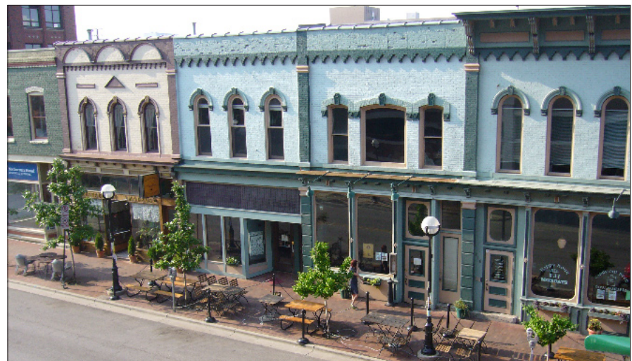
A parapet block refers to a block of buildings with a roof profile that results from being built directly against each other.
