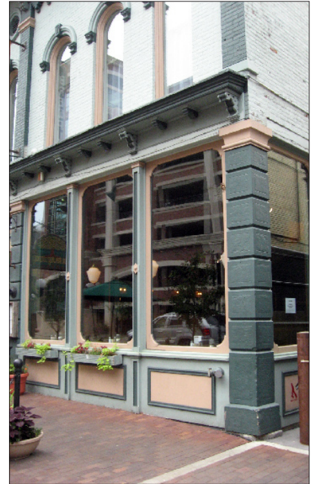
Transparency is the relationship of a building's solid exterior walls to its open or glass areas.
