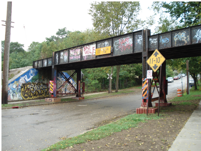
Figure 25: Northern segment of the railway elevated.
