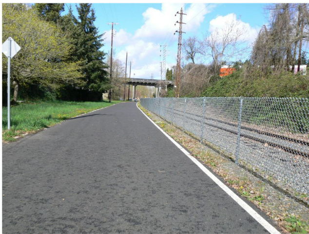
Figure 11: Separation of a greenway from railroad tracks by fence
