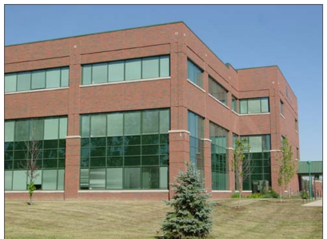
Multiple story office buildings can reduce imperviousness
