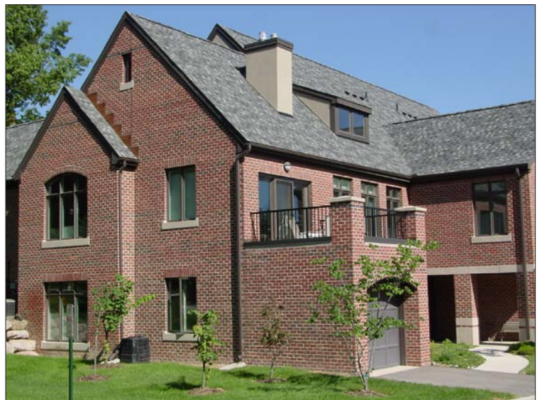
Private residential open space above a garage.
