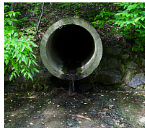
Storm sewer outlet
