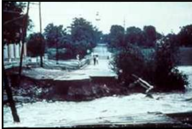
The '68 Dixboro Bridge Wash Out. Source: The City of Ann Arbor, June 2005
