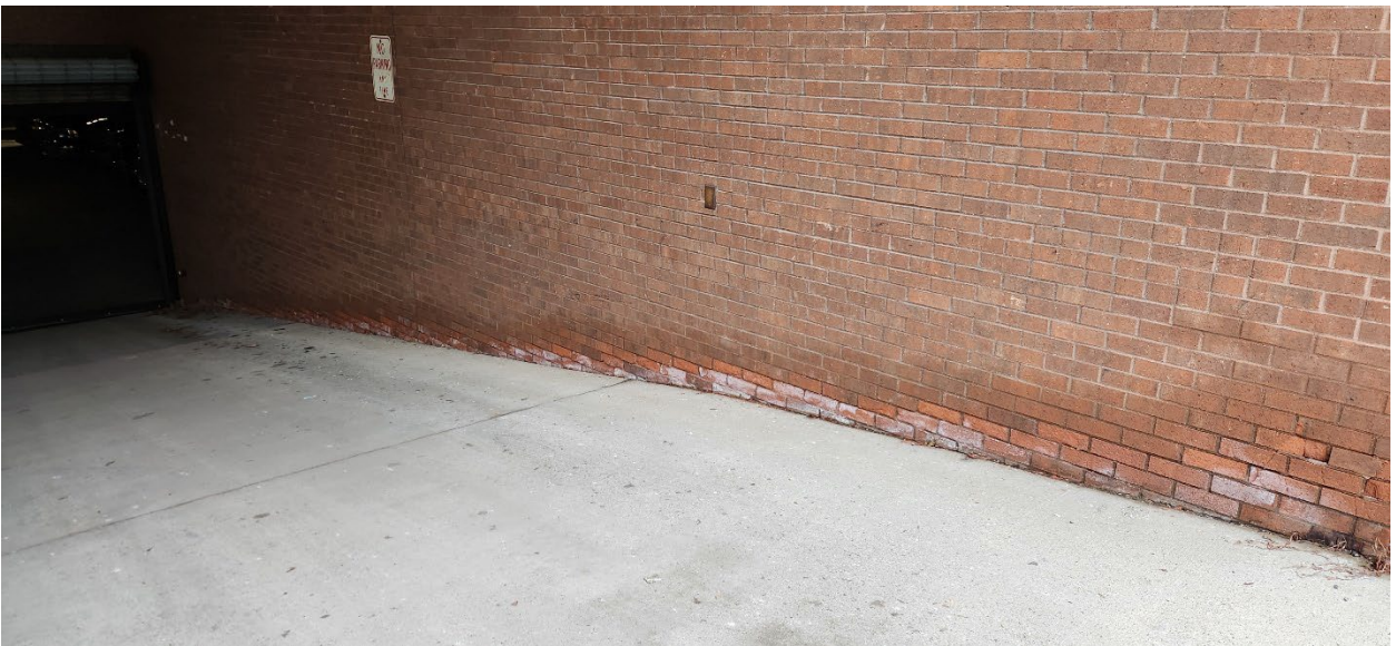
(above) Ann St – west wall to parking deck
