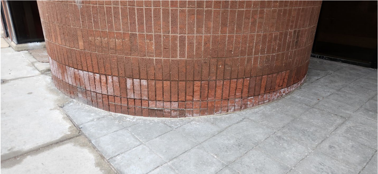
(above) Fifth Ave – area outside elevator shaft
