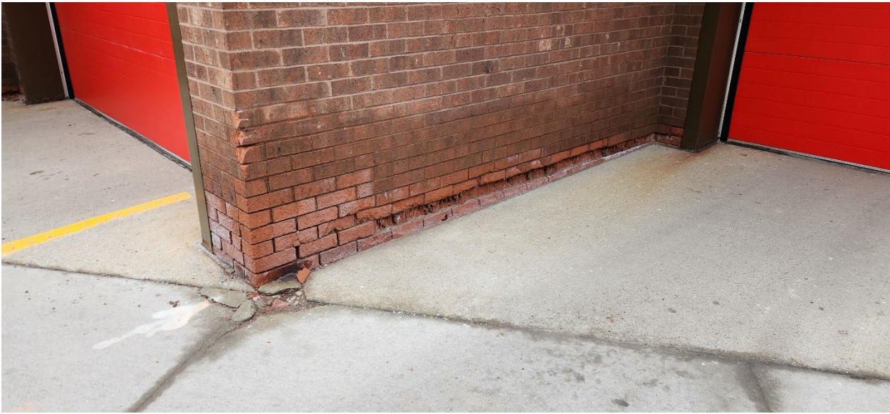
(above) Fifth Ave – wall between bay 4 and 3
