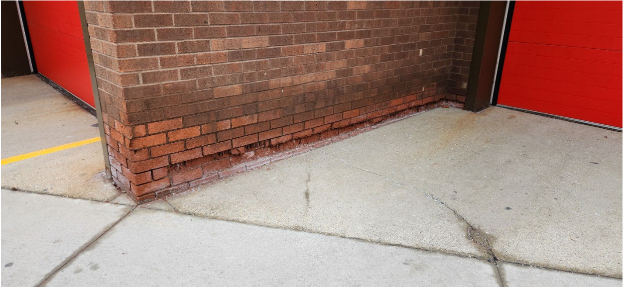
(above) Fifth Ave – wall between bay 7 and 6
