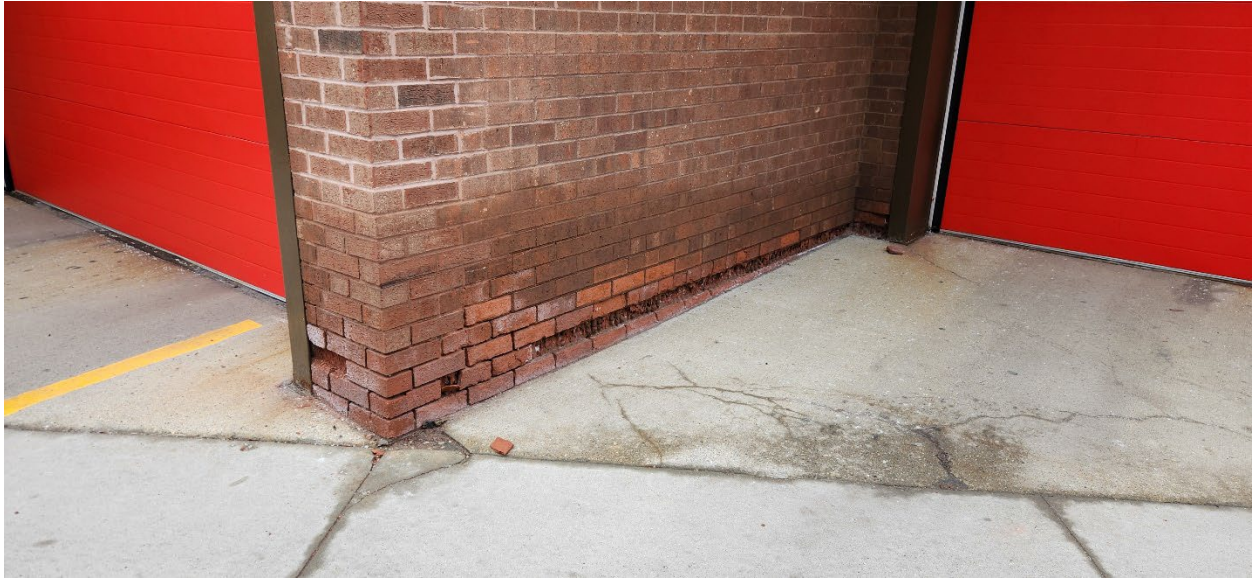
(above) Fifth Ave – wall between bay 3 and 2
