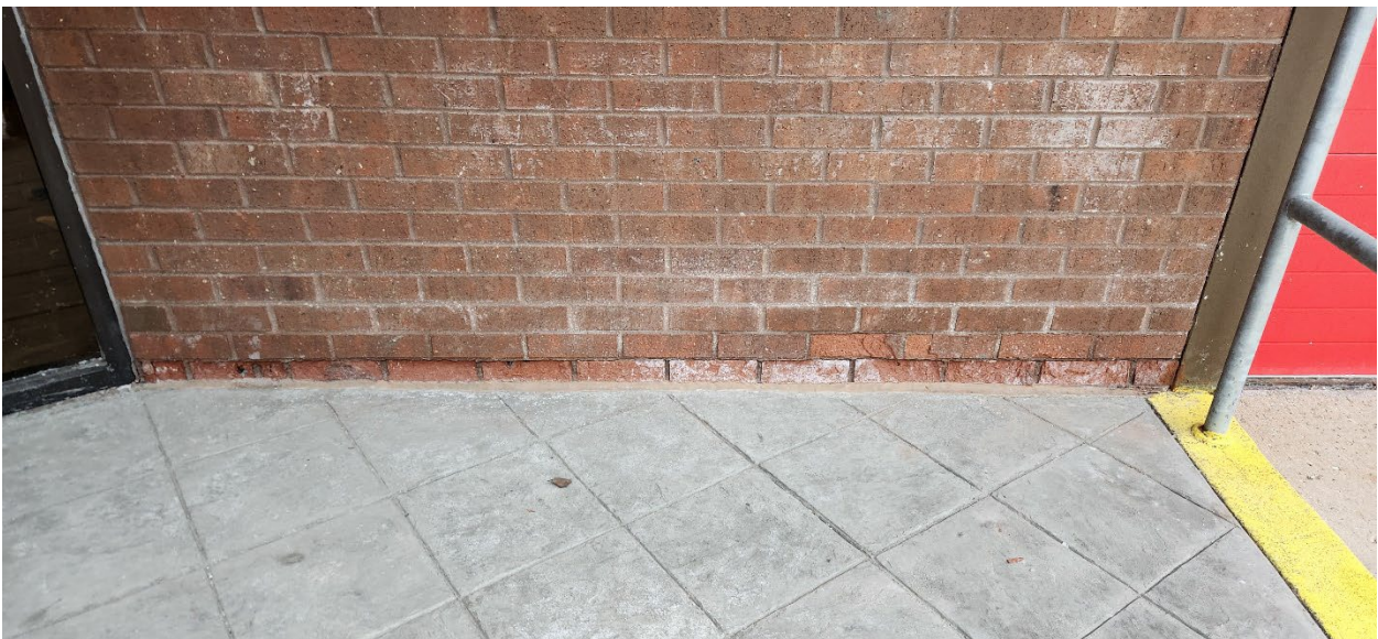
(above) Fifth Ave – area between south entrance door and bay 7
