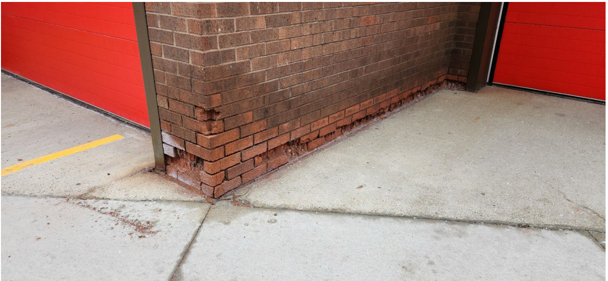
(above) Fifth Ave – wall between bay 6 and 5
