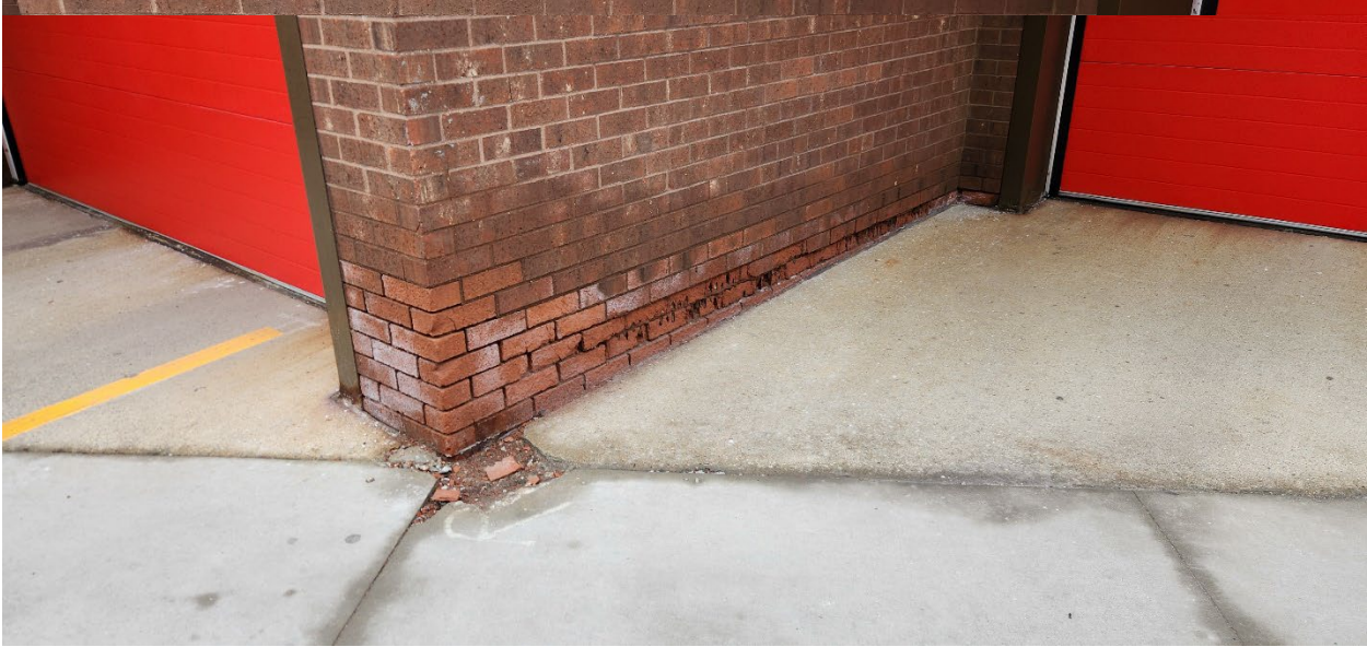
(above) Fifth Ave – wall between bay 5 and 4
