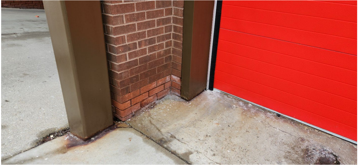
(above) Ann St – outside of bay 1
